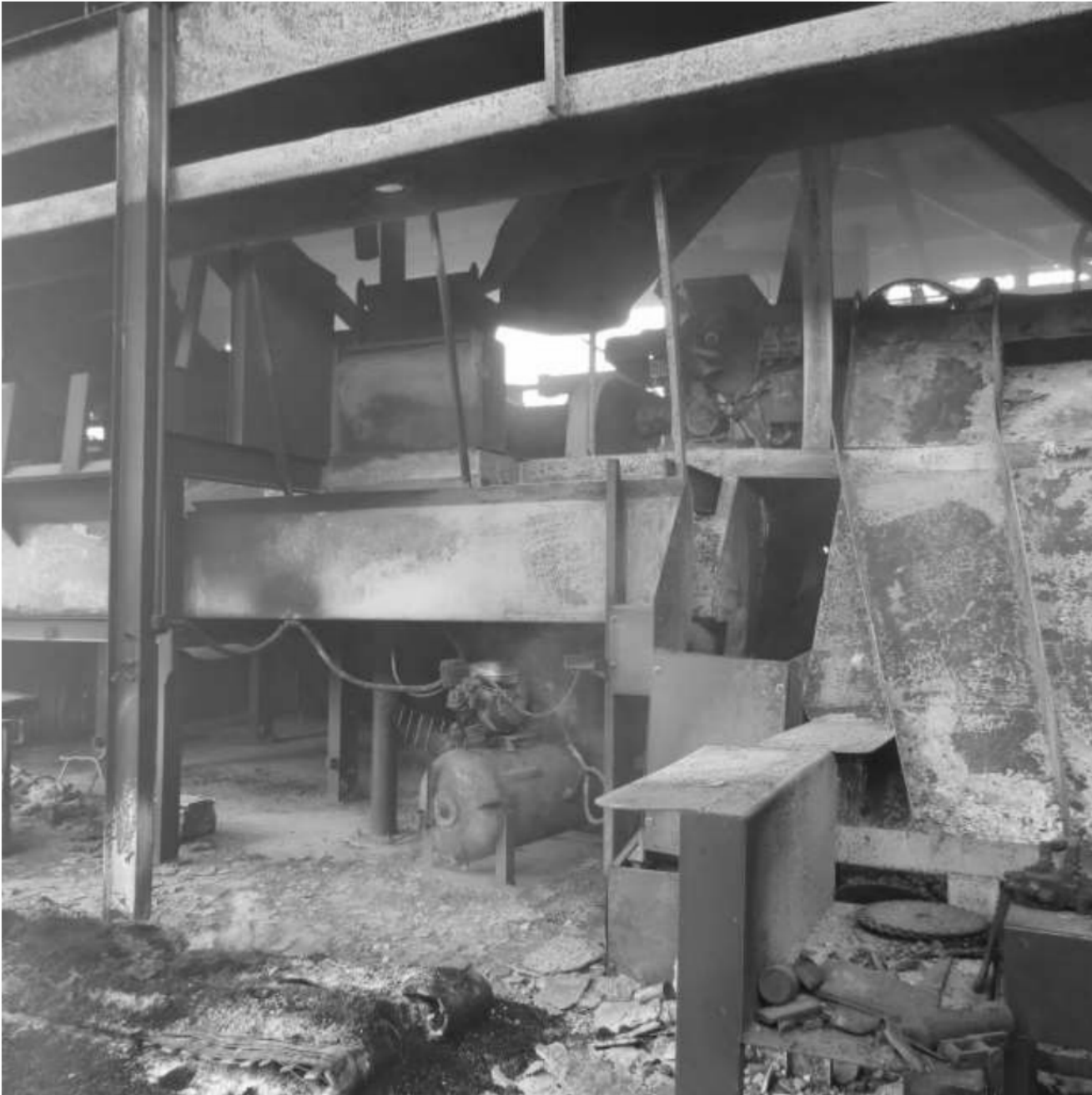
Photo #14 Another example of heat damage to both lower and upper decks & equipment.
