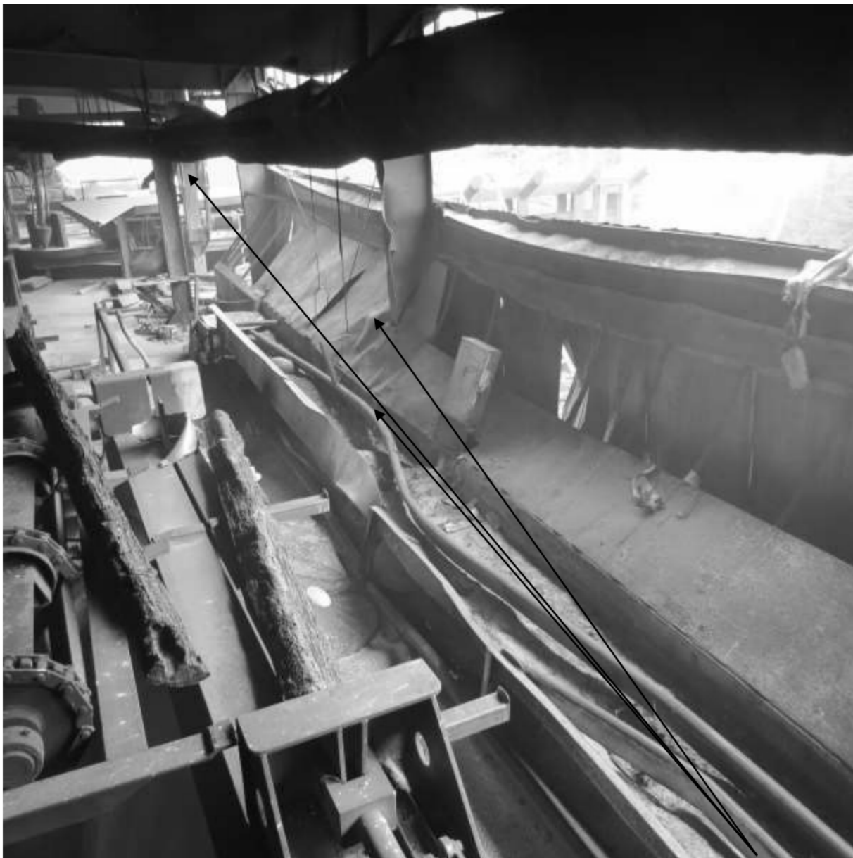
Photo #17 Area above Hydraulic oil tank/electric motors/pumps. High heat- metal buckling
