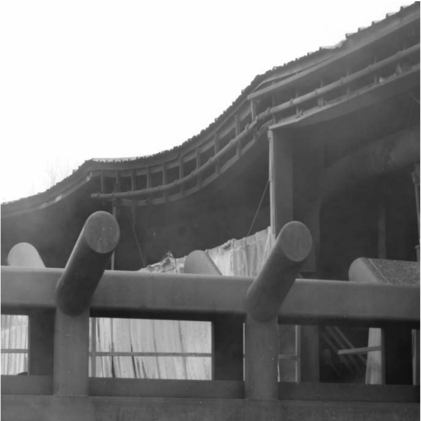
Photo #6 Roof line damage above area of origin which was on grade level - this is above 2 nd story - main mill operations floor.
