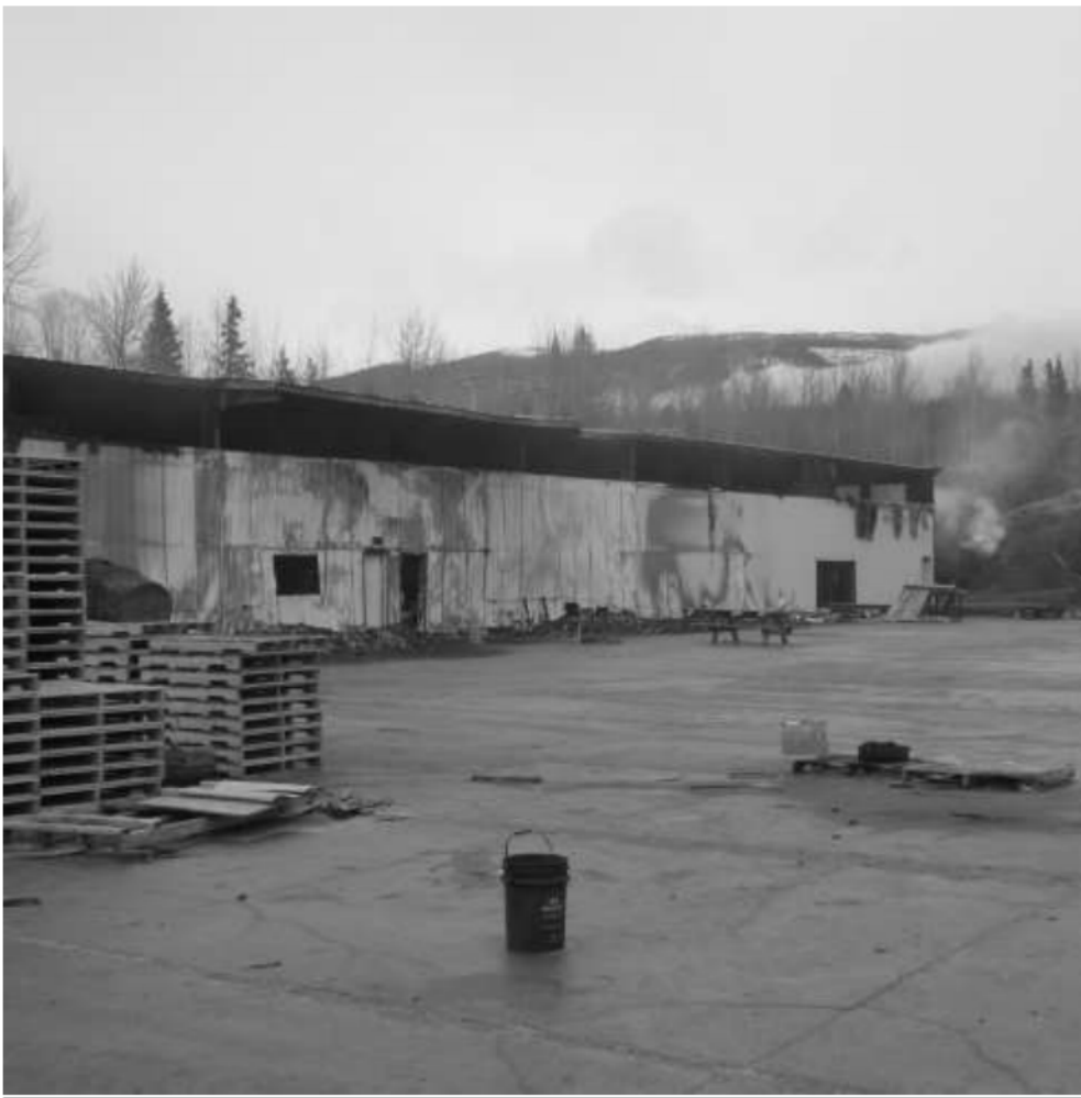
Photo # 1 “A” Side of building - Chip pile to the right is an exposure fire and started after the mill was already burning.
