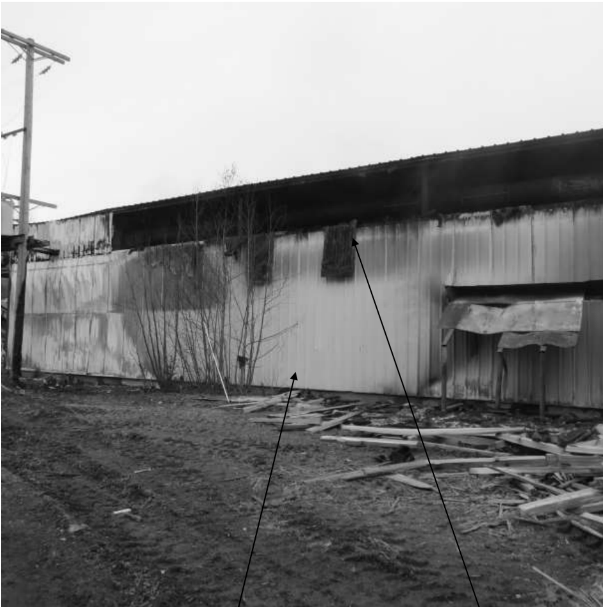
Photo #7 "C" Side of building - Metal cladding. Top row was clear fibreglass to let in natural lighting and in most cases has melted away.
