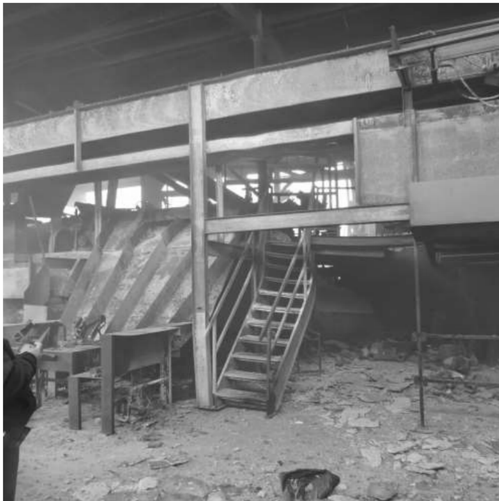
Photo #13 two-thirds the way down looking from D side - Looking towards "C" (back wall) 4 separate stairs going up to main deck - one on each end and two spaced in between the two end stairs.
