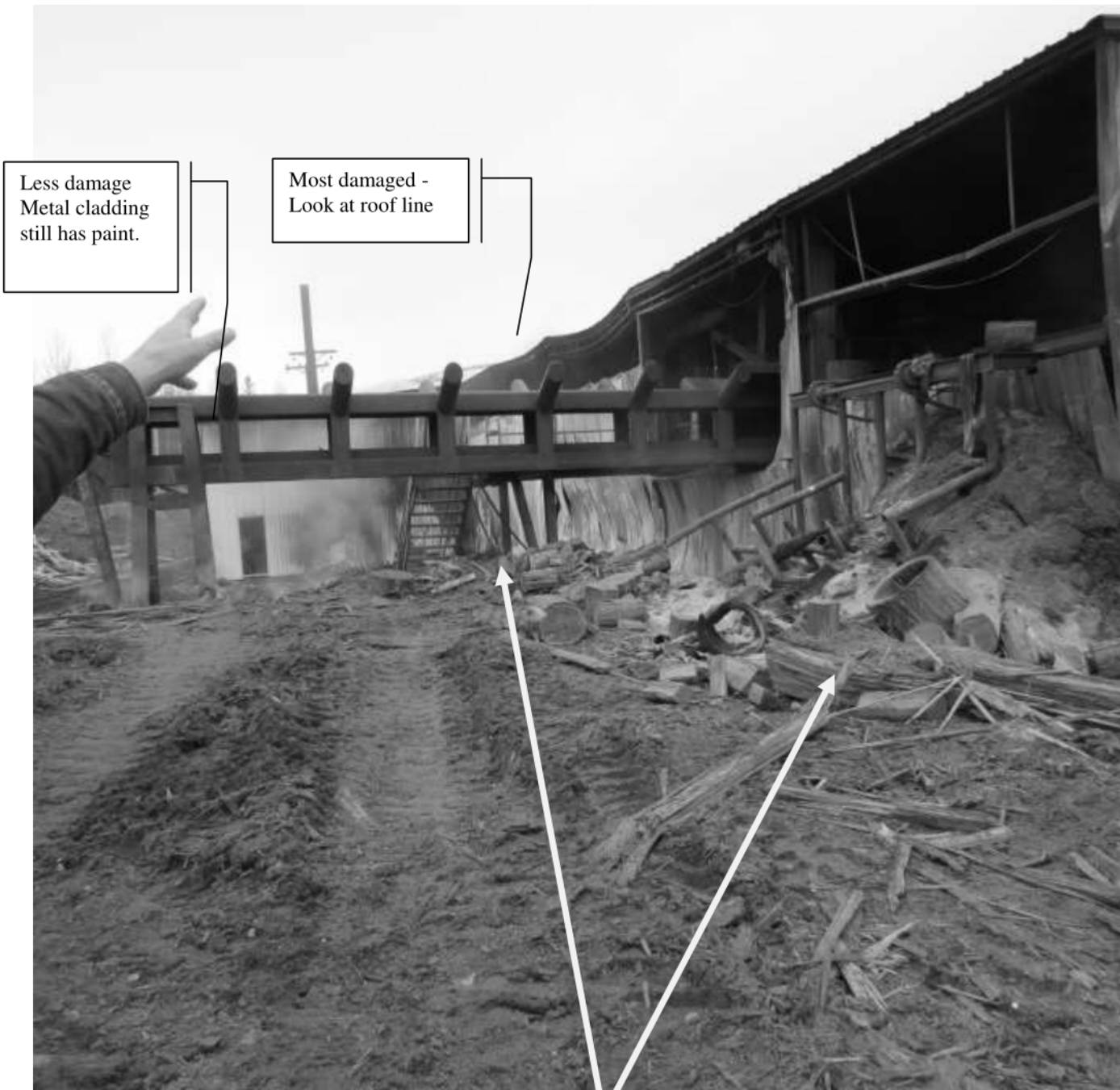
Photo #5 “C” Side of the building (Back) Additional wood on outside of building added to fire load.
