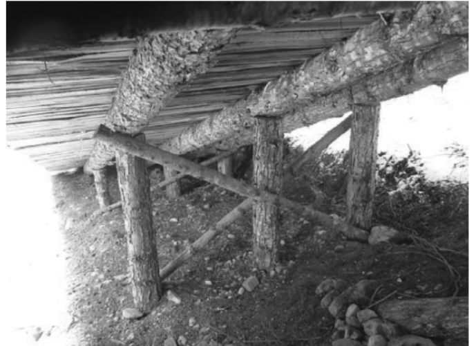
Lower Ramp Posts, Stringers and X-Bracing
