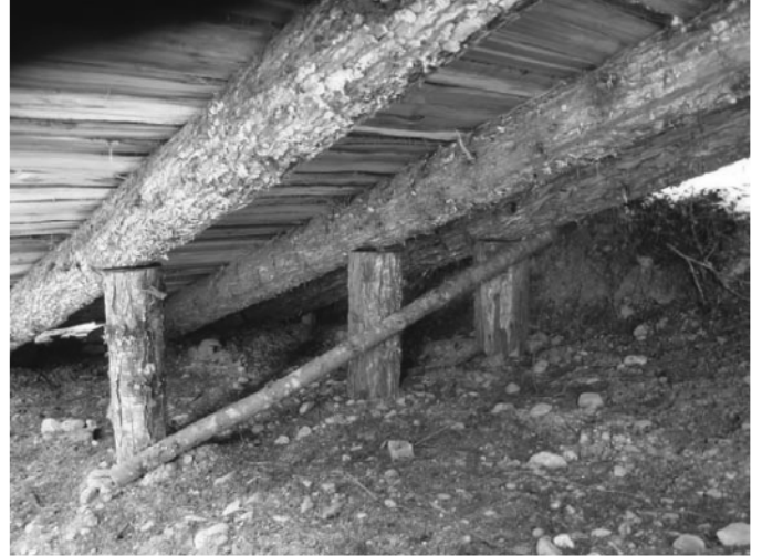
Lower Ramp Posts and X-Bracing
