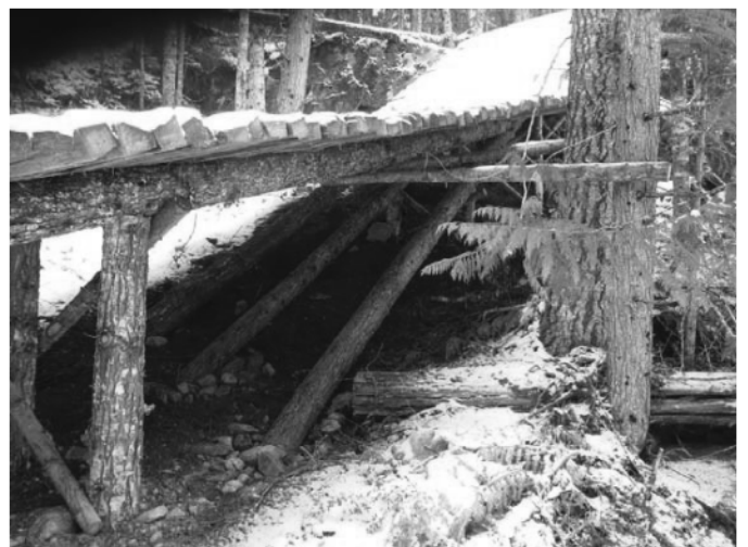
Lower Ramp X-Bracing attached to Trees
