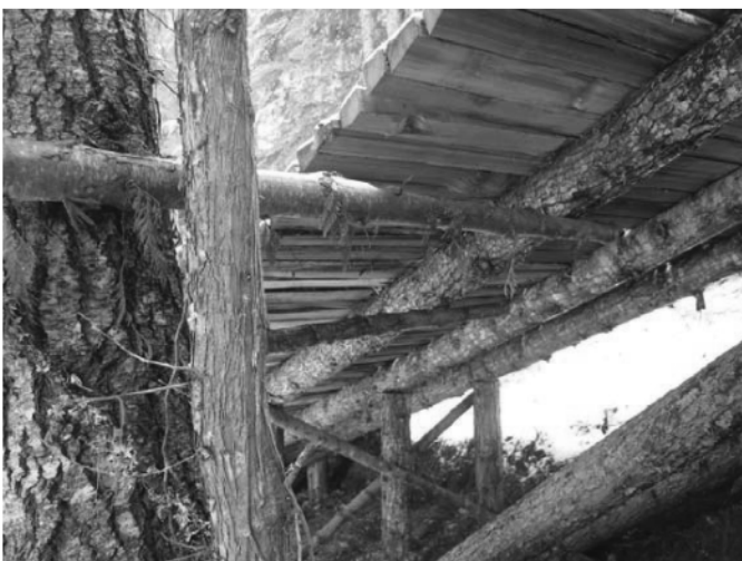
Lower Ramp X-Bracing and Anchor to Tree
