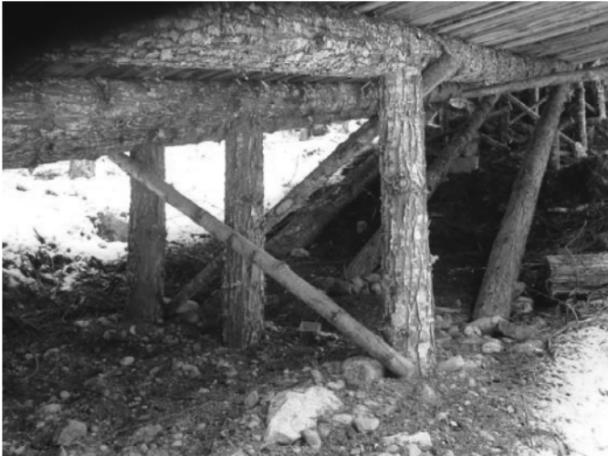
Lower Ramp Posts with X-Bracing Upper Ramp Stringers
