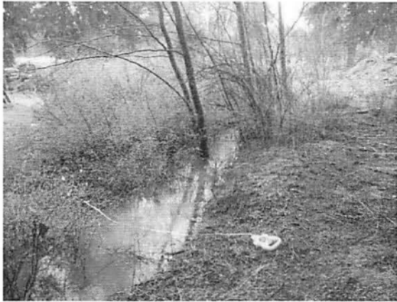
Photo 3-4. View upstream (south) of the roadside ditch along Timberlane Road (above left). Note turbid water in ditch resulting from runoff through active construction site on Lot A (above right). Recommendations for check dam install to mitigate sediment laden water leaving the site have been made and are expected to be installed in the near future.
