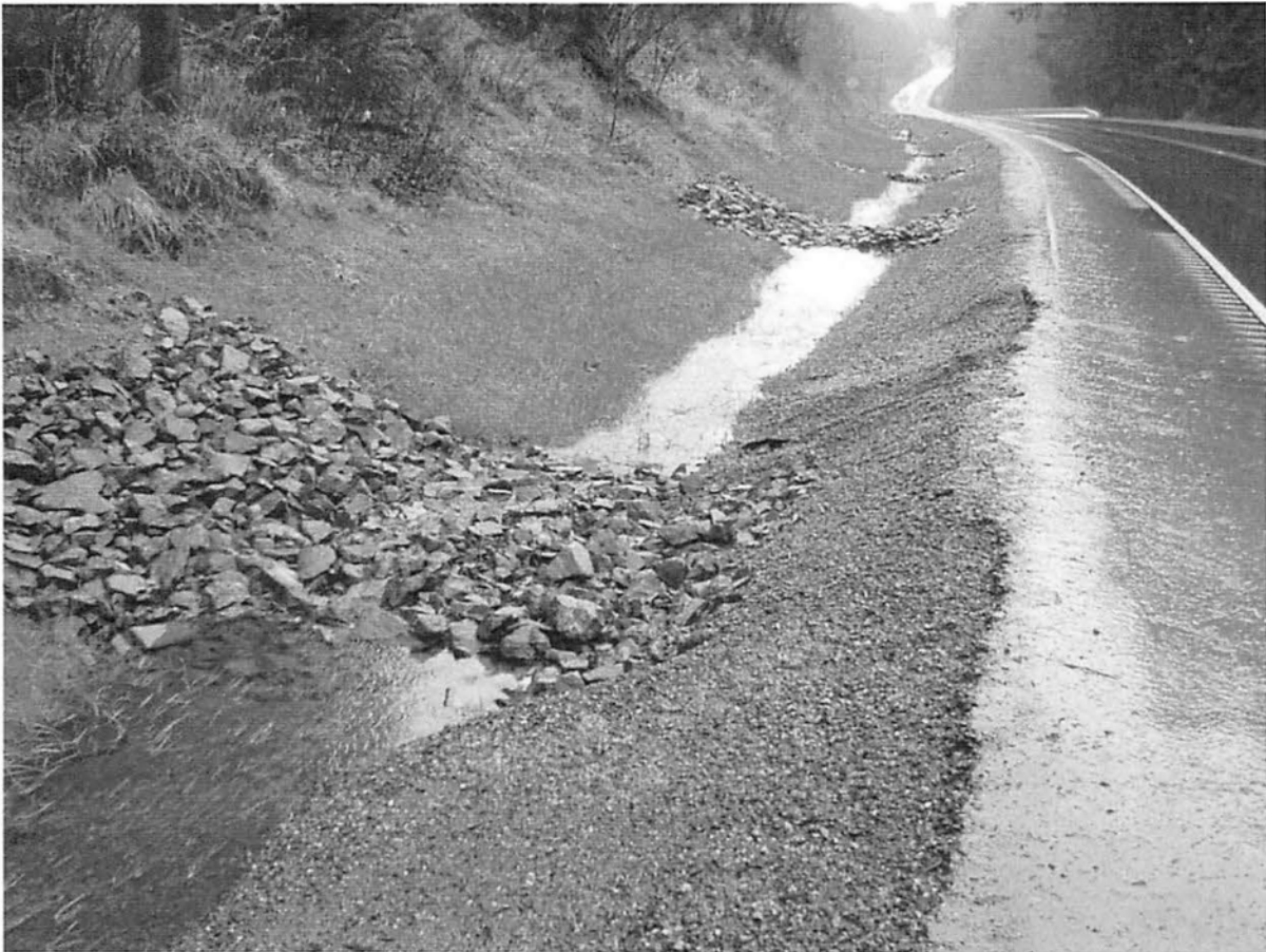
Photo 1. View downstream of appropriate rock check dams used to filter sediment and reduce flow velocities.
