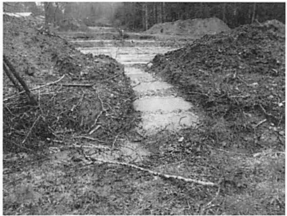
Photo 3-4. View upstream (south) of the roadside ditch along Timberlane Road (above left). Note turbid water in ditch resulting from runoff through active construction site on Lot A (above right). Recommendations for check dam install to mitigate sediment laden water leaving the site have been made and are expected to be installed in the near future.
