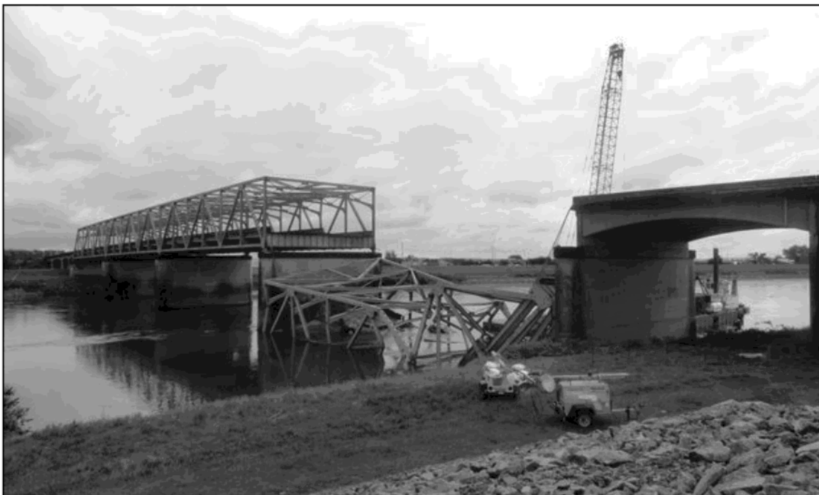
FIGURE 3: SKAGIT RIVER BRIDGE
