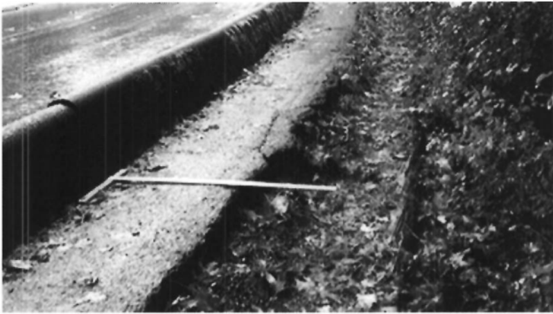
Figure 4: 'Sidewalk' width along route less than 3/4 meters with abrupt edge. Extensive debris
