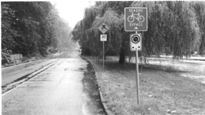
Figure 1: NW Marine Drive along Spanish Banks – Usage and Speed Signage, Lane Width, No Shoulder, Large Puddle forcing cyclists into mid-laneway
