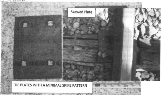
The statement above is correct but not complete. As per the Photo above when rail is spiked, spikes are applied opposite to each other, this prevents the plate from "skewing". However, if the tie on which the plate sits is in poor condition or if there are surface issues at that location, the spike is lifts out or breaks and allows the tie plate to skew. There is no misleading here.
