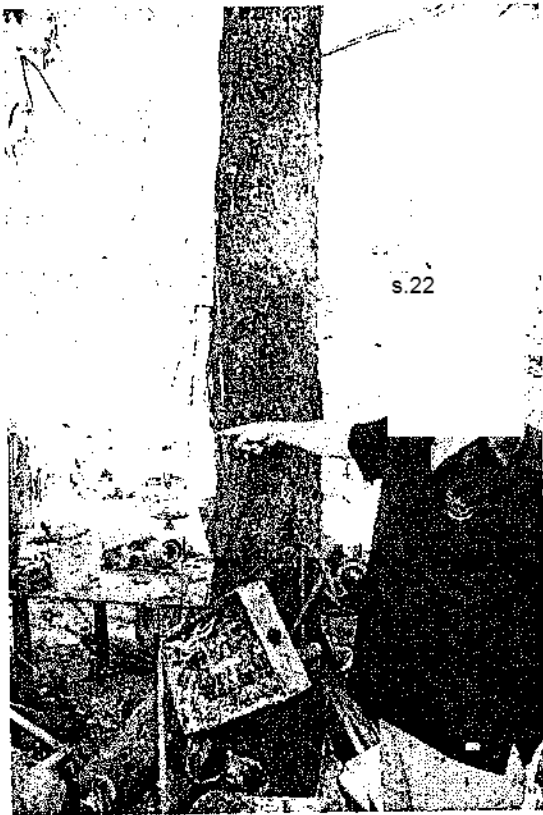
Picture of wires exiting the subpanel and traveling up the tree
