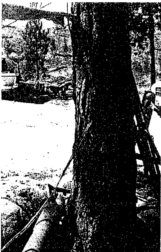
Conductor run down the tree into the ground
