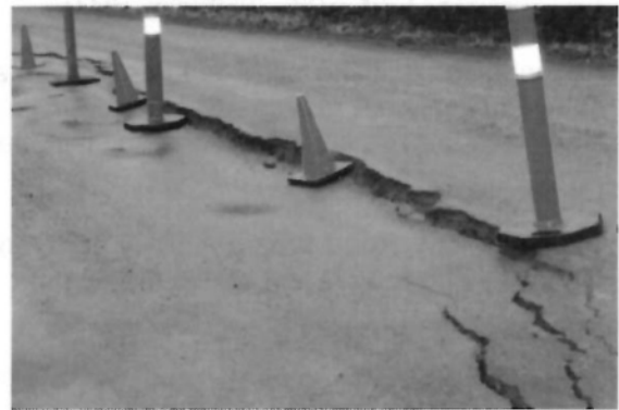
Photo 2: Vertical offset of crack
