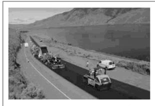
Hot-in-place recycle paving produces **50% fewer greenhouse gas emissions** than conventional paving, as it reuses and recycles existing material, right at the project site.
