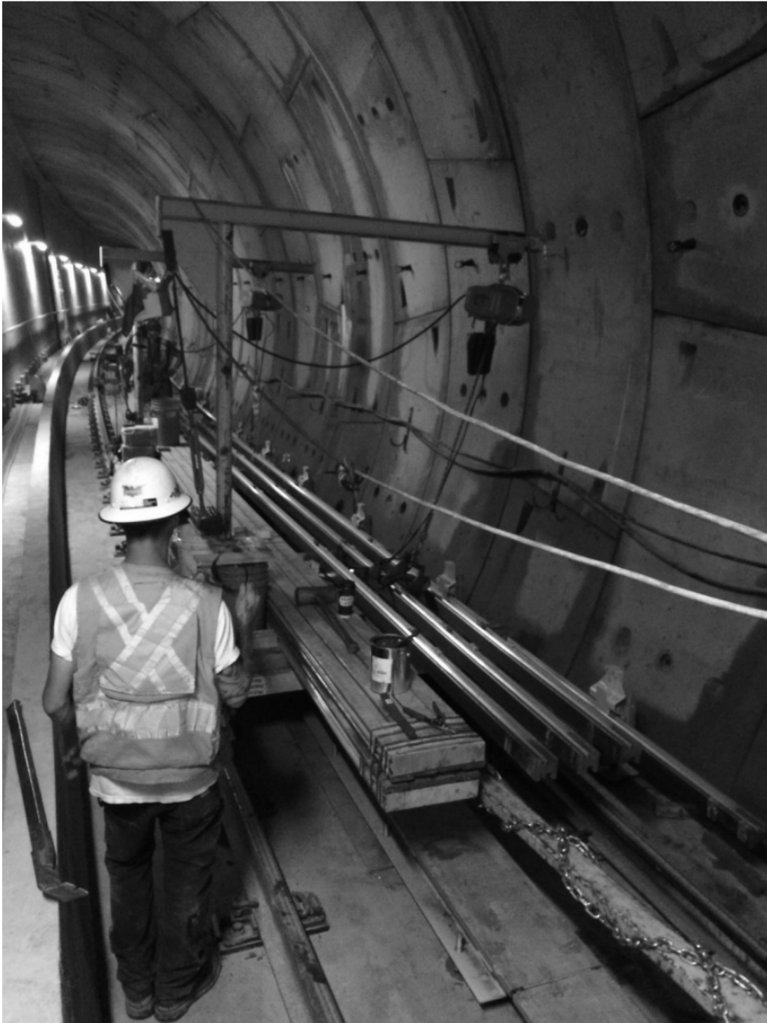
Figure 2 – Power Rail Offloading and Installation
