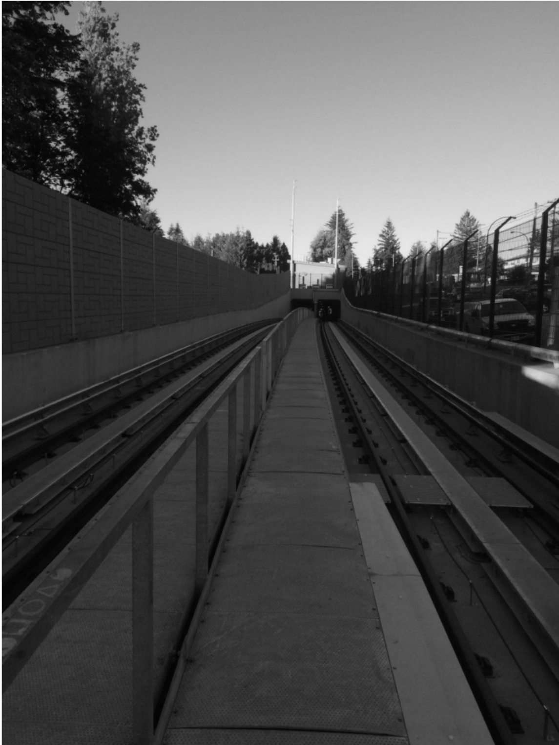
Figure 3 – Completed Walkway installation at South Portal Transition
