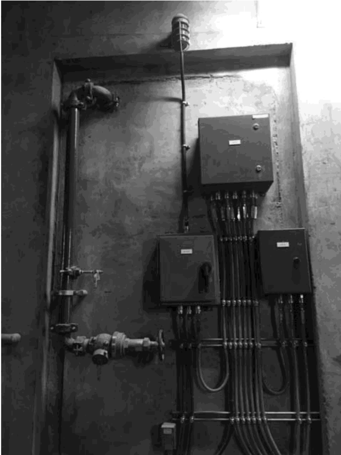
Figure 3 – Cross-passage Blue light station, ETEL and FLSS connection panel
