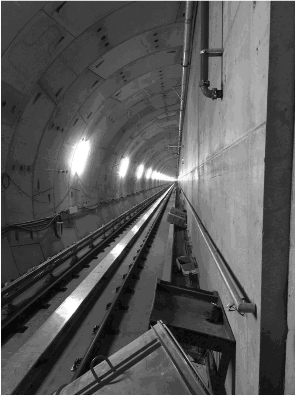
Figure 1 – Main Rail, LIM Rail, and Power Rail Completed Portion in Inbound Tunnel
