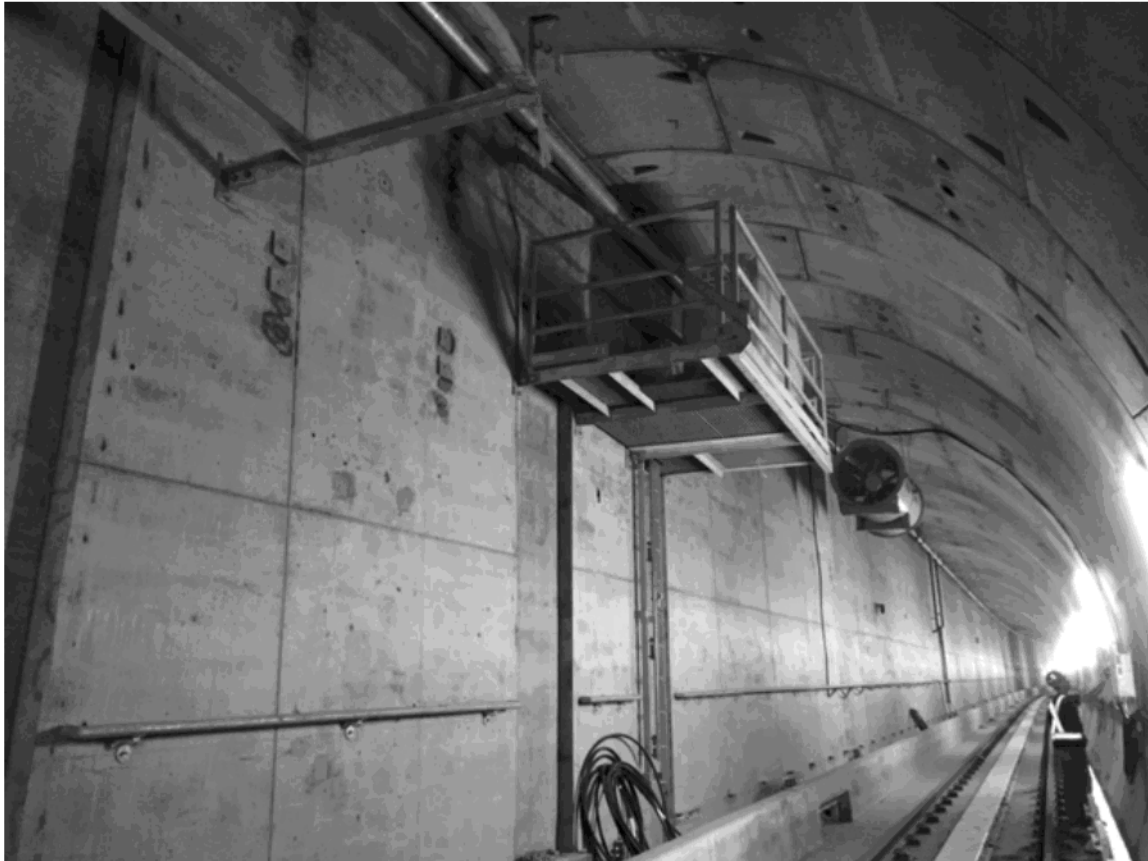
Figure 5 – Tunnel Inbound Propulsion Power Disconnect Switch Platform
