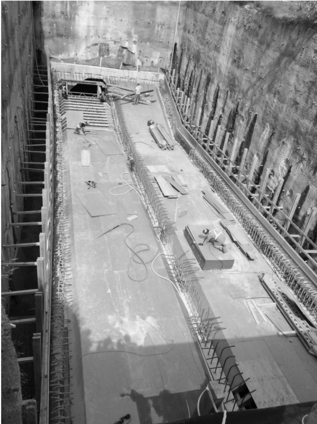
Figure 1 – Formwork in Preparation of South Portal Transition Pour
