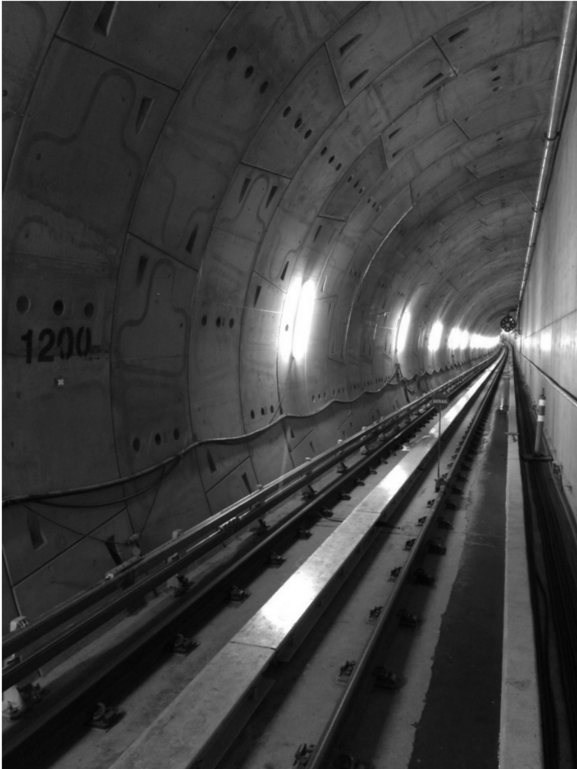
Figure 3 – Tunnel Section with completed Running Rail, LIM and Power Rail
