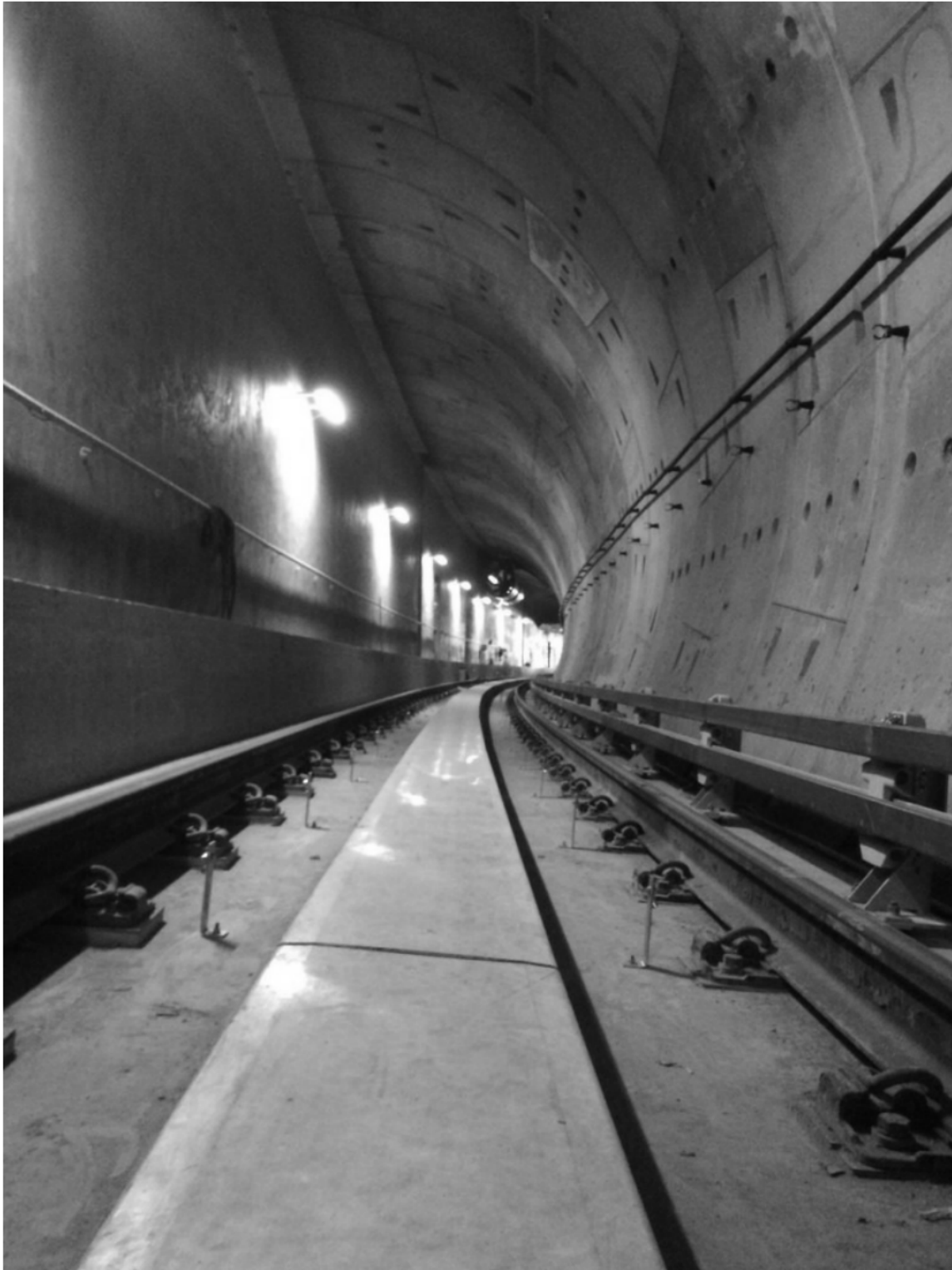
Figure 3 – Completed LIM/Power/Running Rail on OB Track
