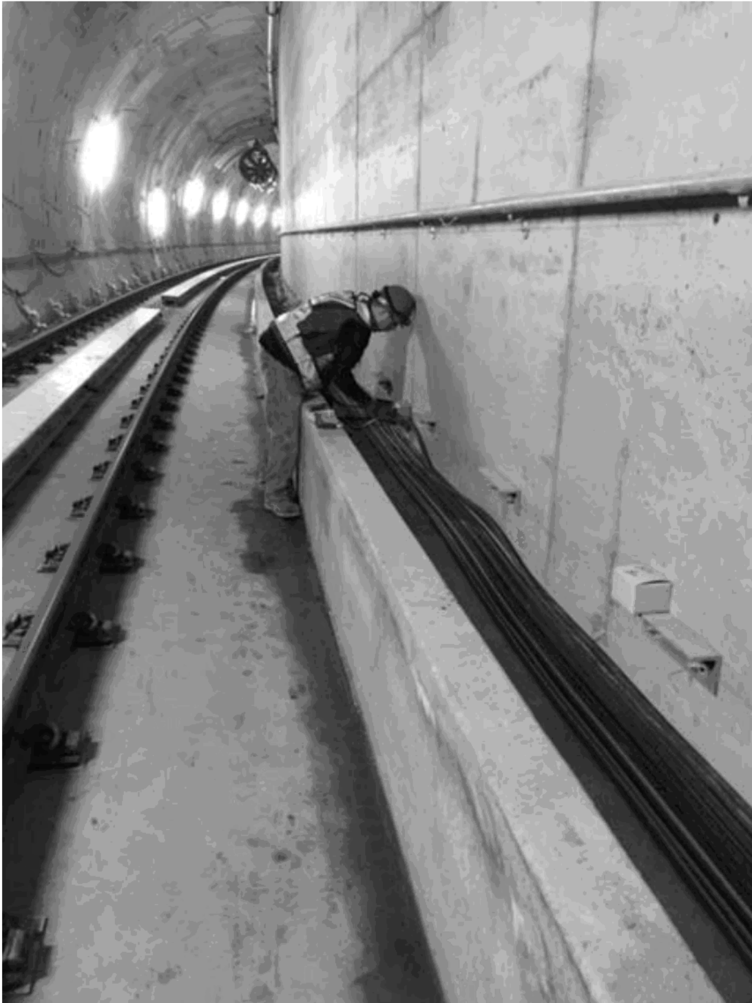
Figure 2 – Lighting feeder junction box installation
