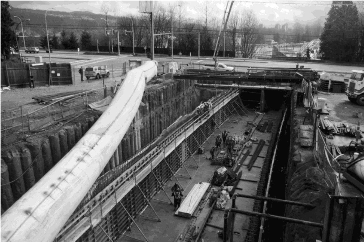
Slab and walls to North Portal cut and cover tunnel are under construction
