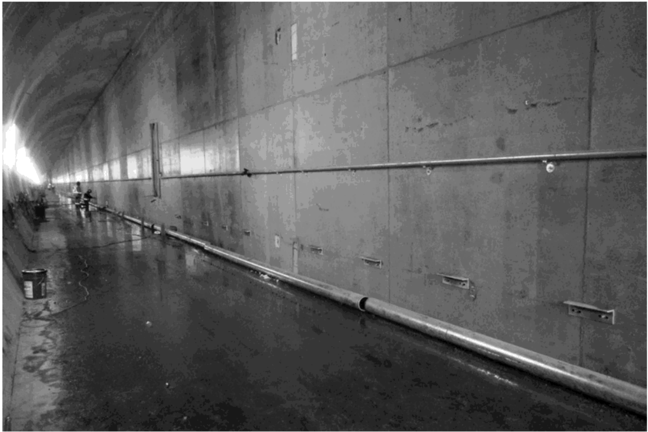
Installation of handrail, firemain and walkway brackets started on dividing wall.
