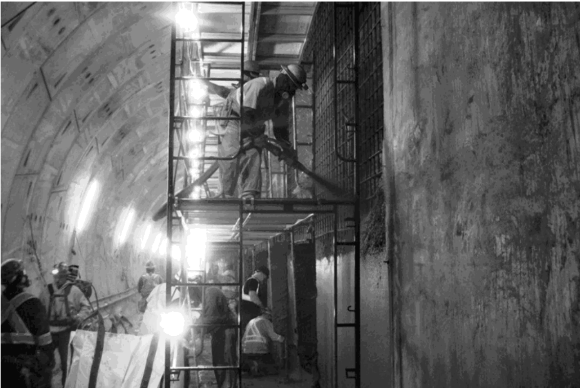
Structural shotcrete of the dividing wall in the tunnel started.
