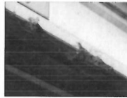
Filename: 01550 132 Girder 2A_impact damage in the bottom flange near north intermediate diaphragm 20140617.JPG
