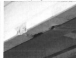
Filename: 01550 160 Girder 2M_impact damage in the bottom flange at north intermediate diaphragm 20140617.JPG
