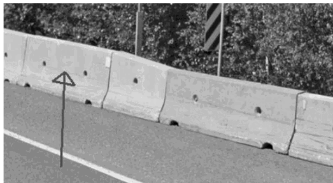
Figure 8 - XSP – G – 810mm (32") New Style Concrete Barrier – with Lifting Holes
