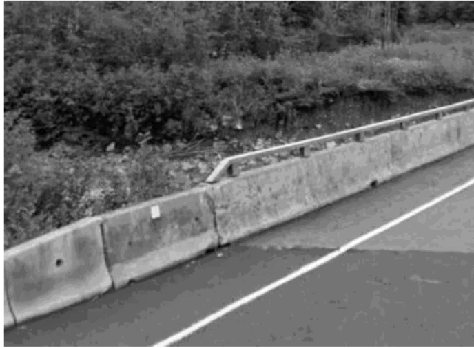
Figure 4 - XSP – C – 760mm (30") Old Style Concrete Barrier – no Lifting Holes
