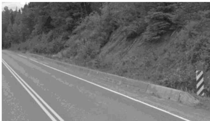
Figure 3 - XSP – B – 460mm (18”) Old Style Concrete Barrier – no Lifting Holes
