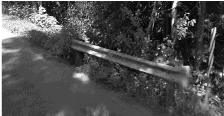
Figure 5 - XSP – D – Sub Standard W-Beam
