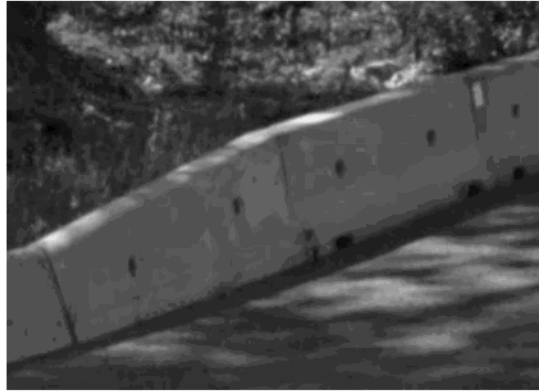
Figure 7 - XSP – F – 690mm (27") New Style Concrete Barrier – with Lifting Holes
