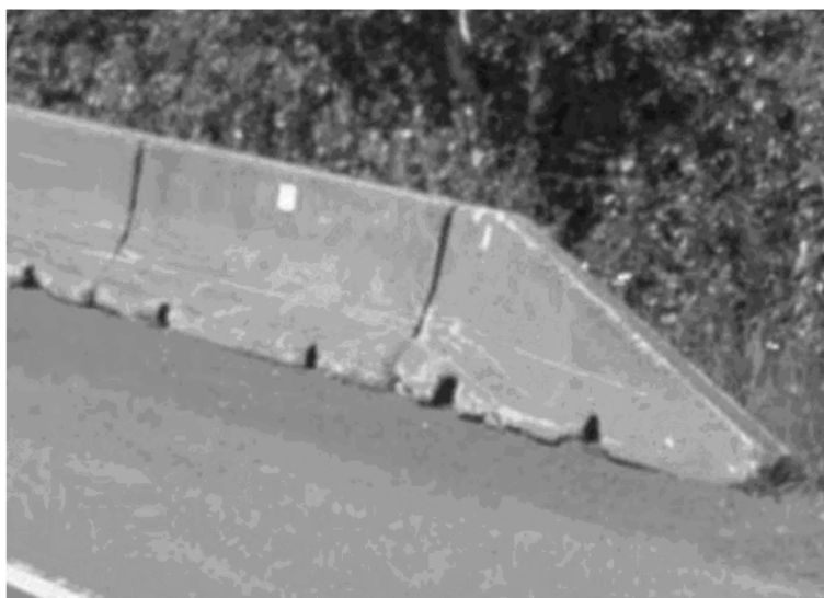
Figure 2 - XSP – A – 690mm (27”) Old Style Concrete Barrier – no Lifting Holes
