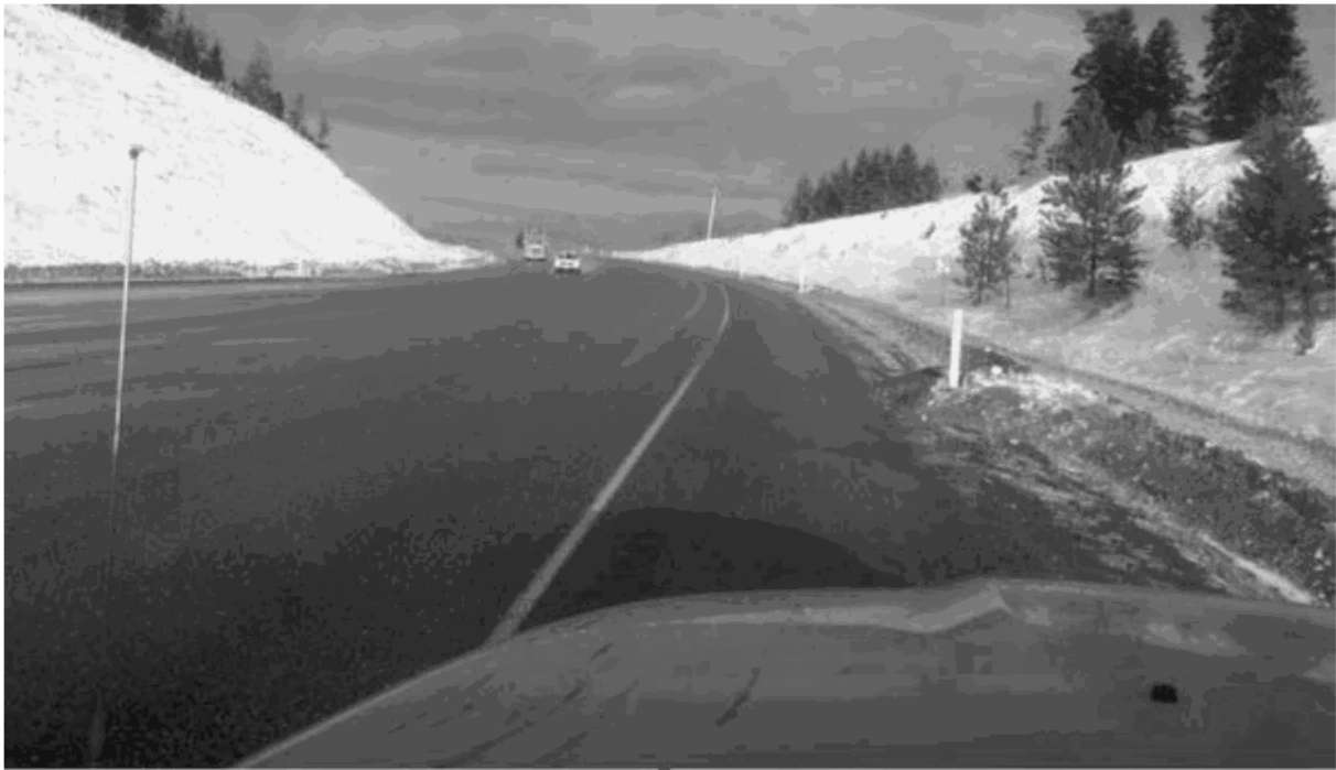
Figure 2 Jan 18 Shldr Grading beyond shoulder side slope Big Bar Hill around delineators
