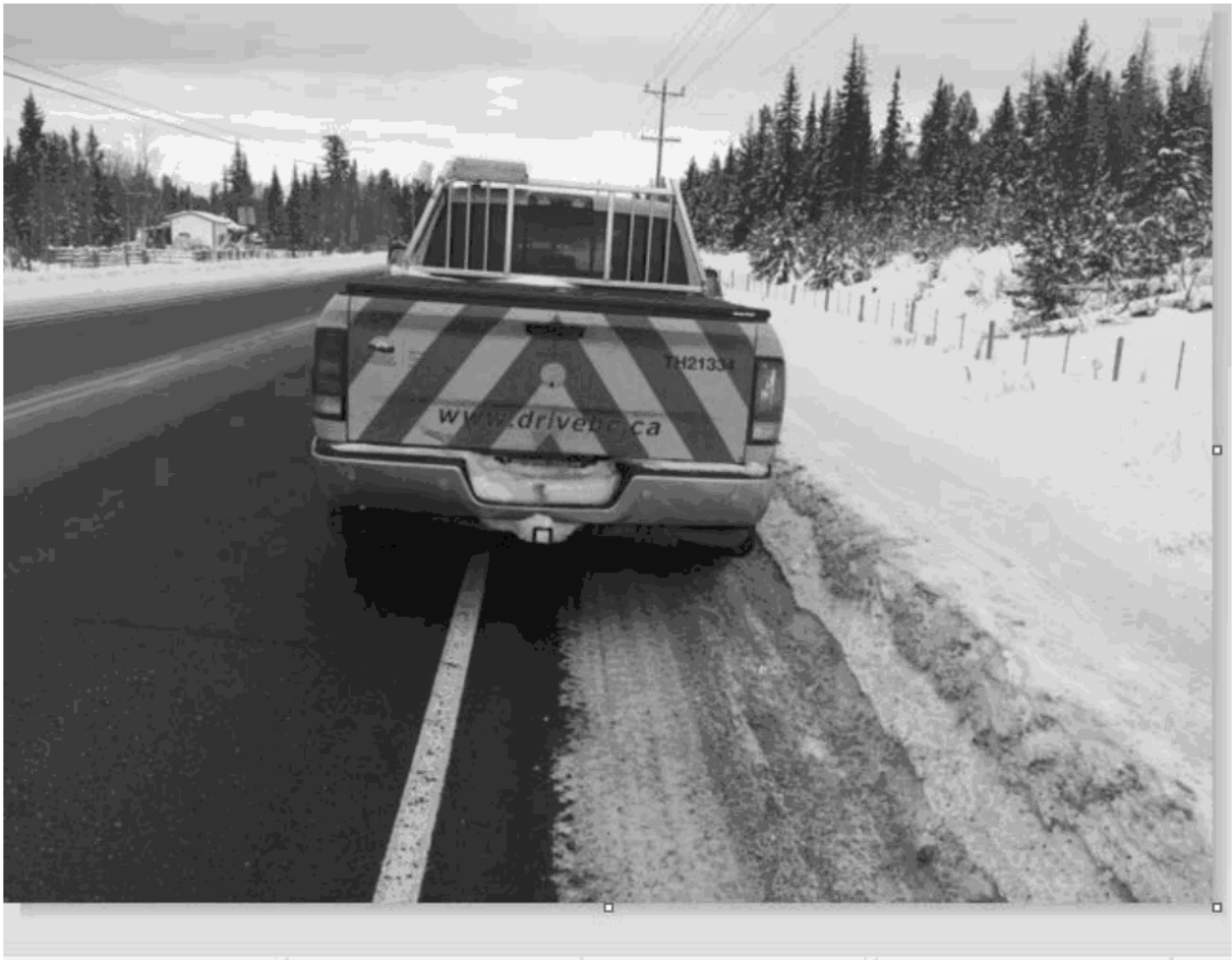
Figure 13 Jan 17 Chasm area - shoulder truck plowed to shoulder edge break line (this is older hwy section & has narrow shoulders)
