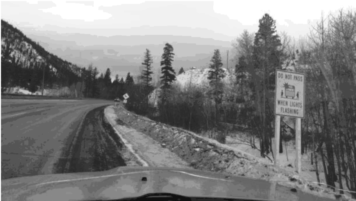
Figure 12 Jan 17 Shoulder grader plowed beyond shoulder side slope to ditch line, signs clean, drains opened
