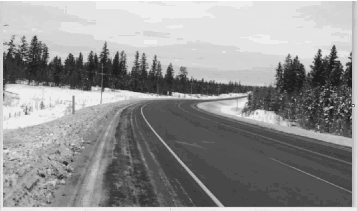
Figure 11 jan 16 plowed to shoulder break point - no meltwater on hwy surface lanes
