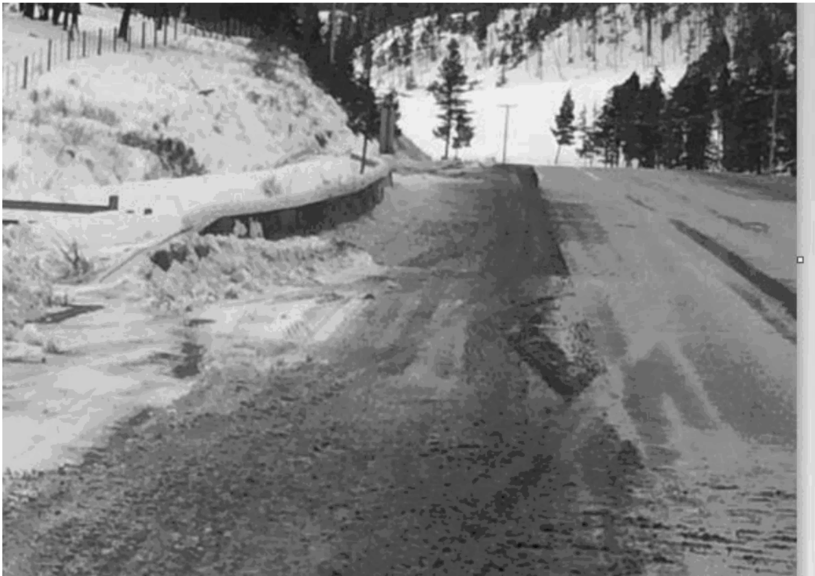
Figure 3 H97 Maiden Creek Hill Jan 17 - Shldr Grading near CRB & drains
