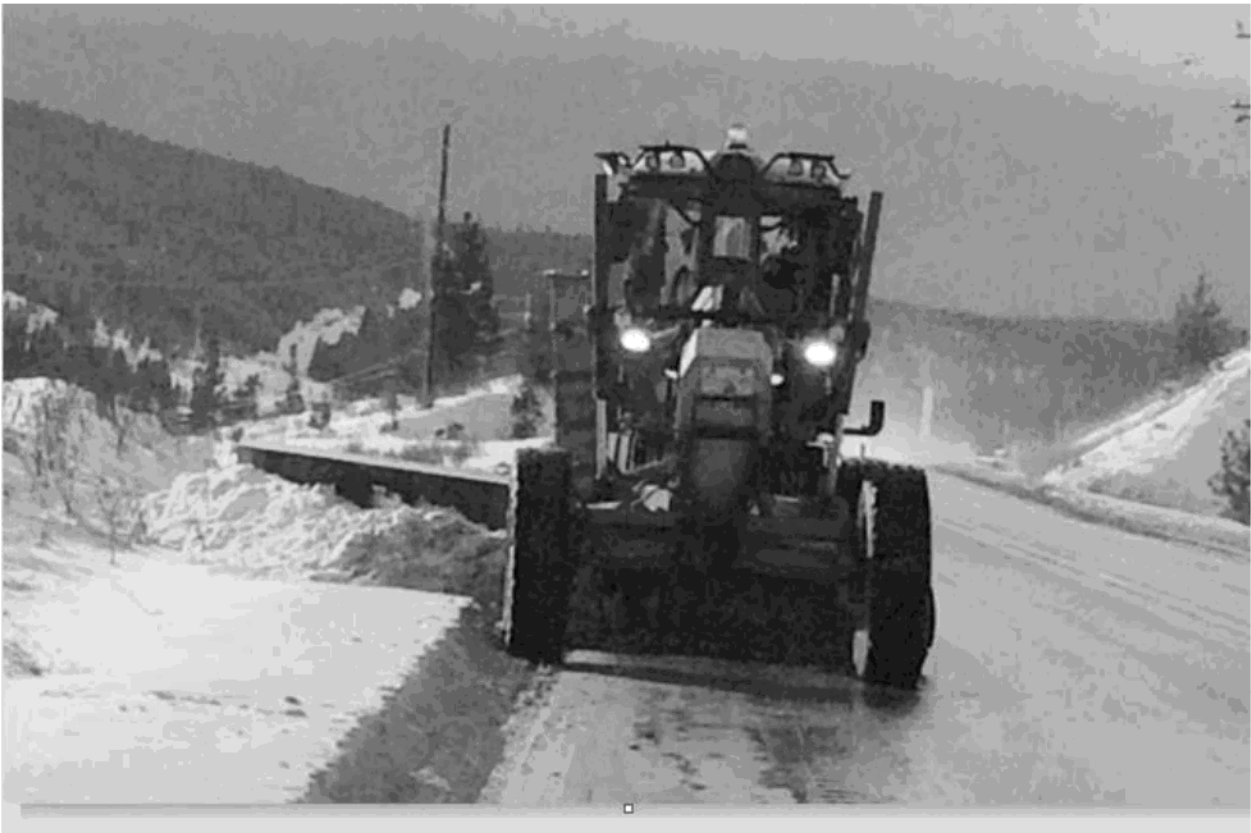
Figure 4 Jan 18 Shldr Grading beyond shoulder side slope and into ditch at Big Bar Hill
