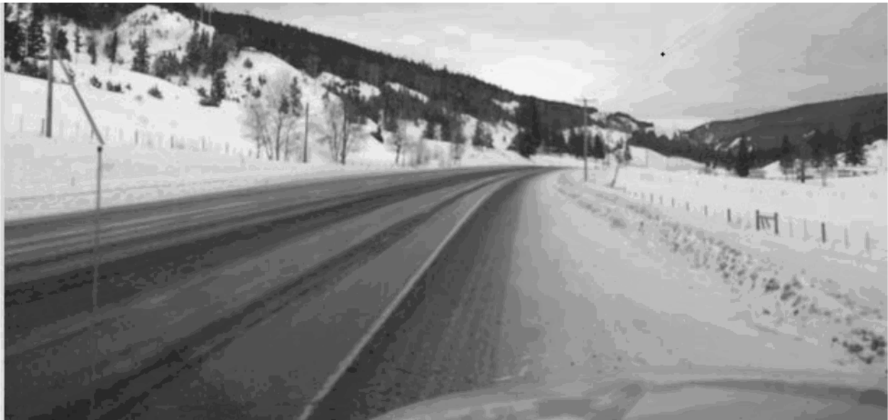
Figure 6 Jan 17 15 km south of Clinton Shldr plowed beyond shoulder side slope to ditch line with grader
