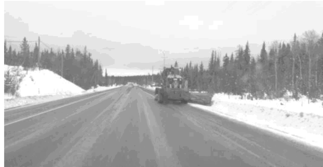
Figure 1 Jan 19 shoulder grading beyond side slope on H97 Chasm area
