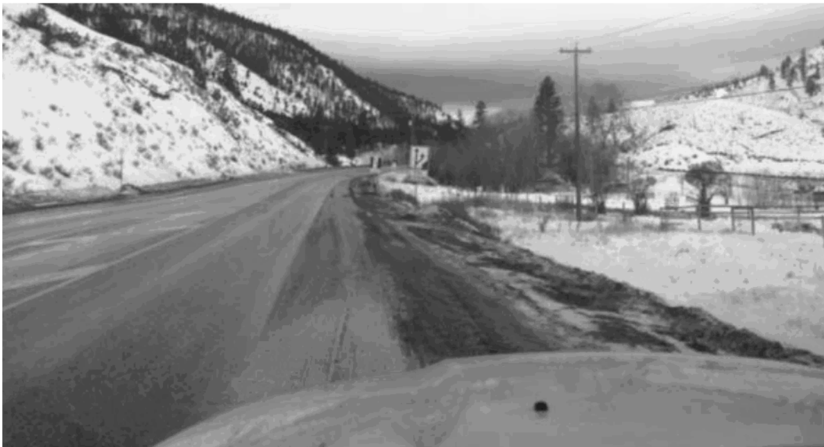
Figure 7 Jan 17 0.2 km north Loon Lake Rd - drains shovelled out, grader shldr plowed beyond shoulder side slope to ditch line
