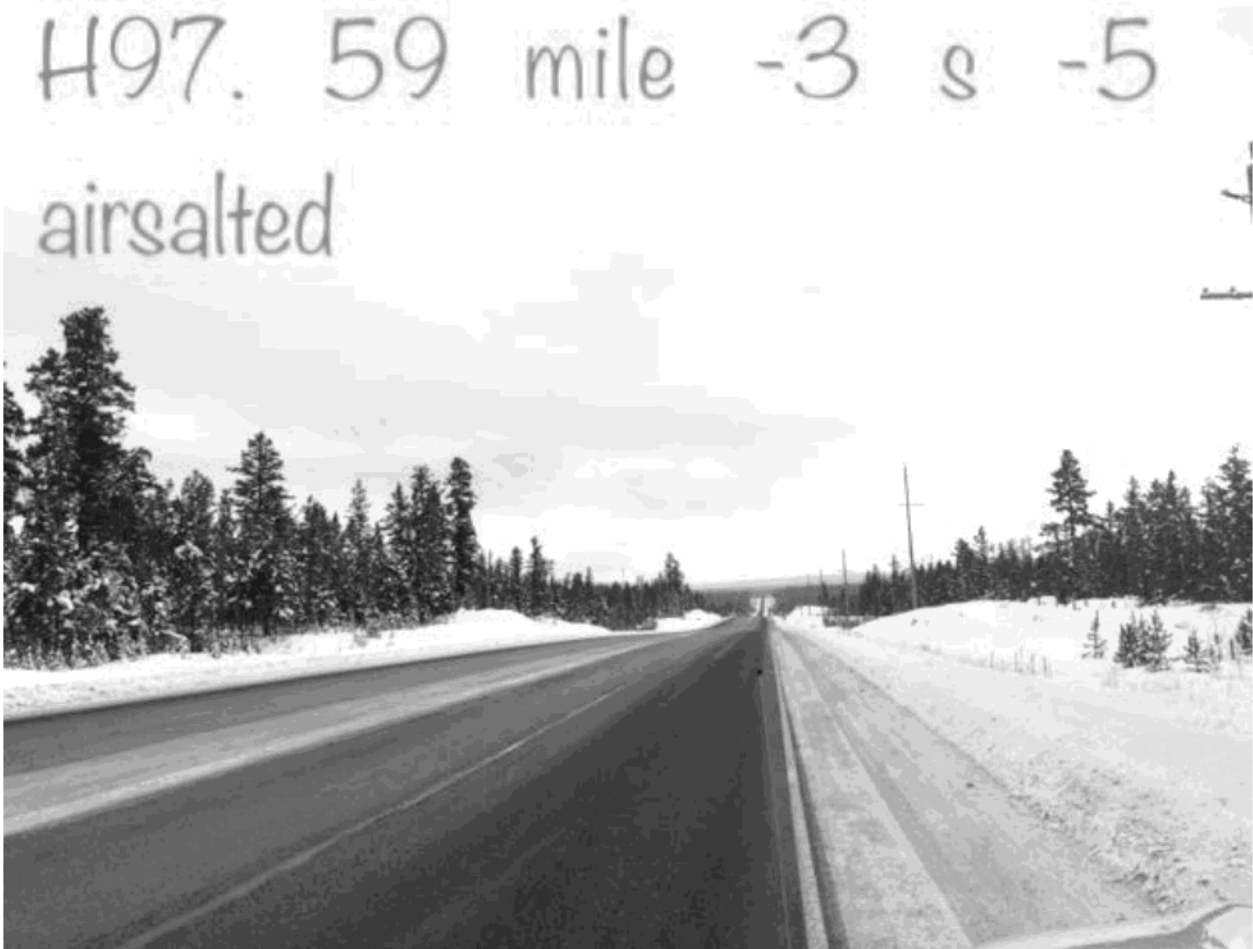
Figure 14 Jan 16 59 Mile truck plowed to shldr edge at break point
