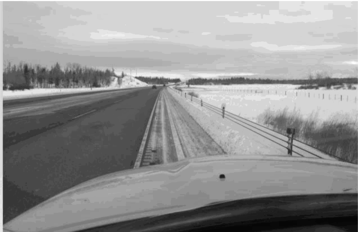
Figure 10 Jan 16 truck plowed to shlder break point at Loch Lomond Cable barrier area
