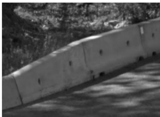
Figure 14 - XSP – F – 690mm (27”) New Style Concrete Barrier – with Lifting Holes
