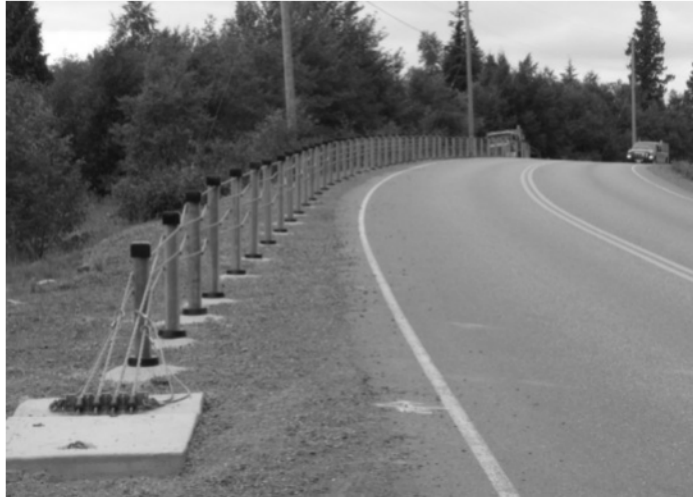
Figure 16 - XSP – H – Cable Barrier
