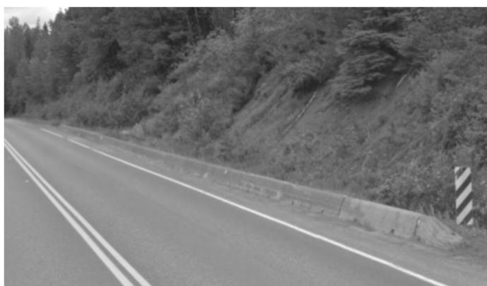
Figure 10 - XSP – B – 460mm (18") Old Style Concrete Barrier – no Lifting Holes
