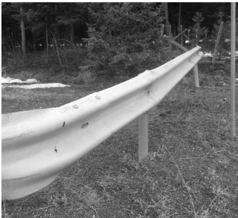
Figure 12 - XSP – D – Sub Standard W-Beam
