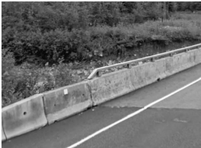
Figure 11 - XSP – C – 760mm (30") Old Style Concrete Barrier – no Lifting Holes
