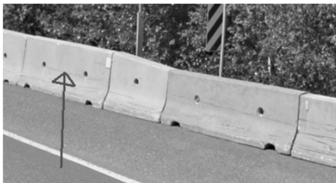
Figure 15 - XSP – G – 810mm (32”) New Style Concrete Barrier – with Lifting Holes
