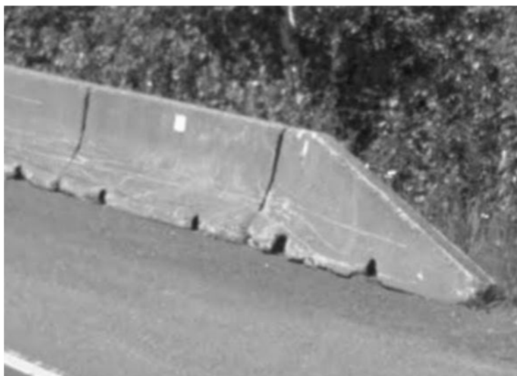
Figure 9 - XSP – A – 690mm (27") Old Style Concrete Barrier – no Lifting Holes
