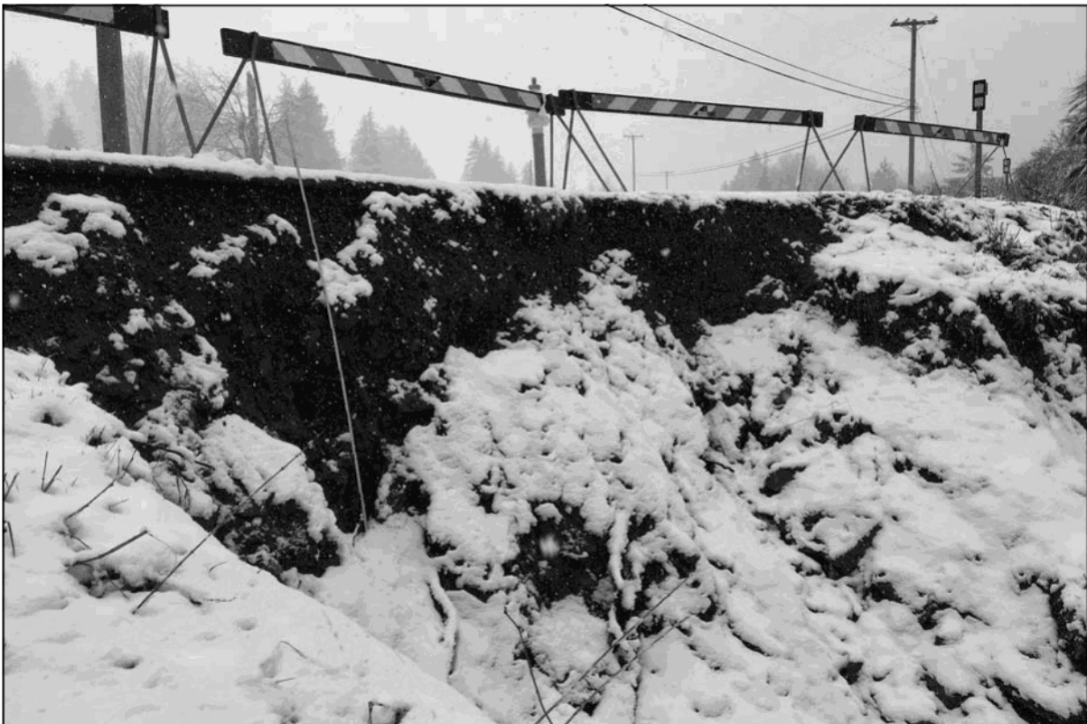
PHOTO 2: View of headscarp of failure. Note ruler is 2.0 m in length.
