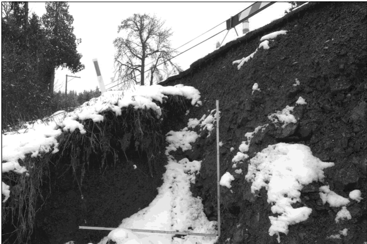
PHOTO 10 View of slump material remaining in place in the failure area.
