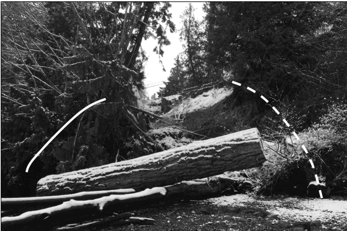
PHOTO 4: View of slide debris from base of slope. The proposed remedial measures involve leaving the large logs and tree in the foreground in place, and constructing the buttress behind this material. The dashed line forms the approximate northern end of the "Full Treatment" and "Minimal Treatment" areas. The solid line forms the approximate southern end of the "Minimal Treatment" area, while the southern end of the "Full Treatment" area is out of frame photo 4 left.
