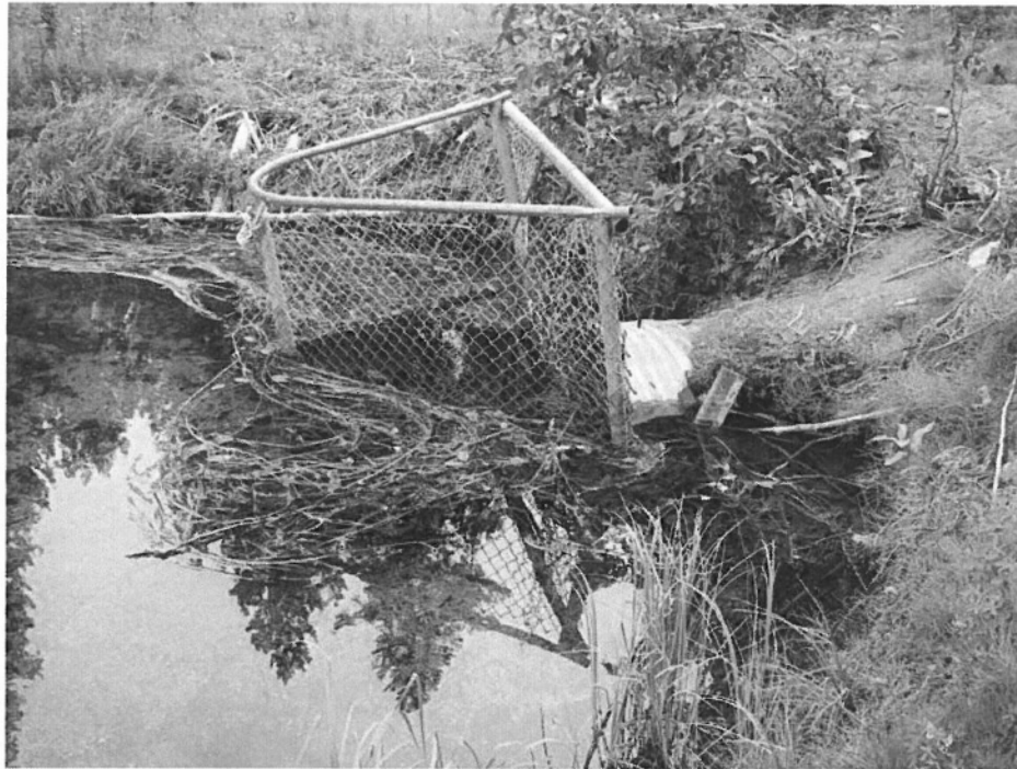
Photo 7: View of culvert with wire grate at the outlet to Lajoie Lake, 20 August 2007.
