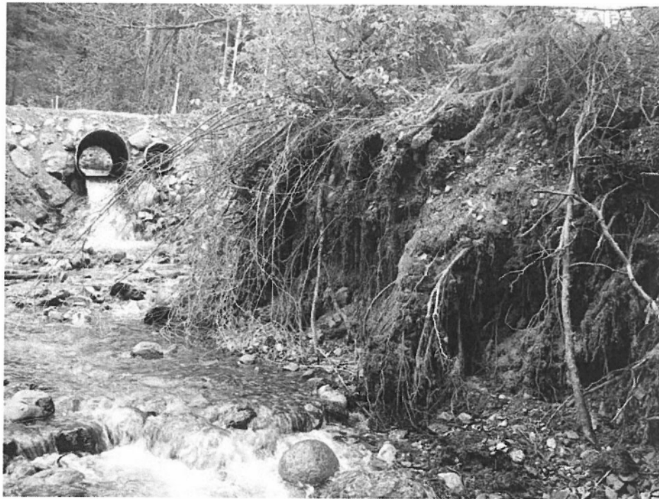
Photo 3: View of eroding left downstream bank downstream of the culvert crossing on Jim Creek, 20 August 2007.
