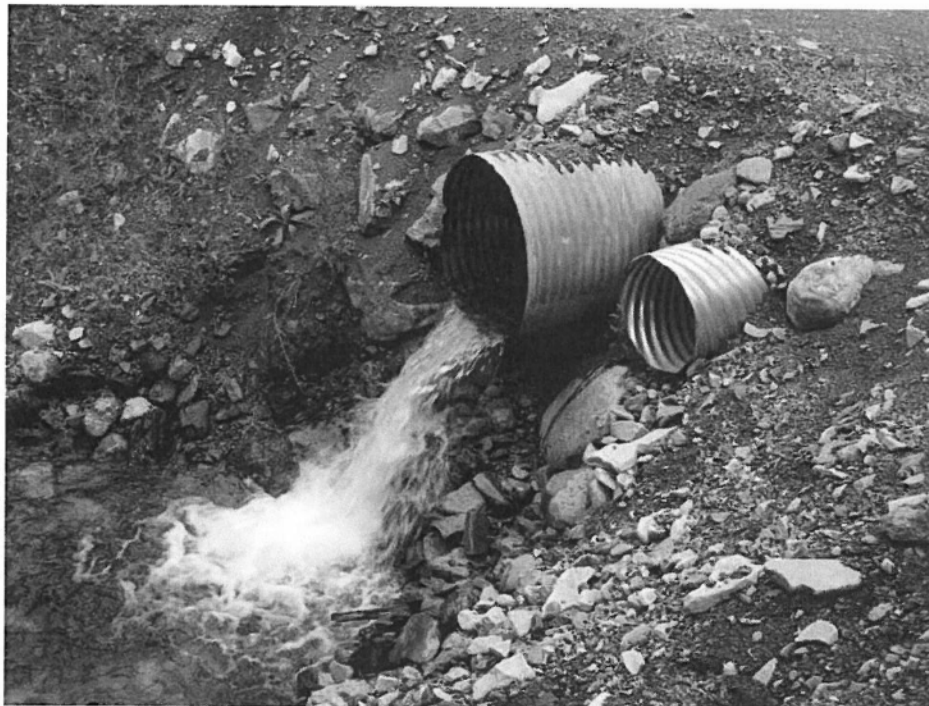
Photo 4: View of hanging culvert at Jim Creek crossing, 20 August 2007.
