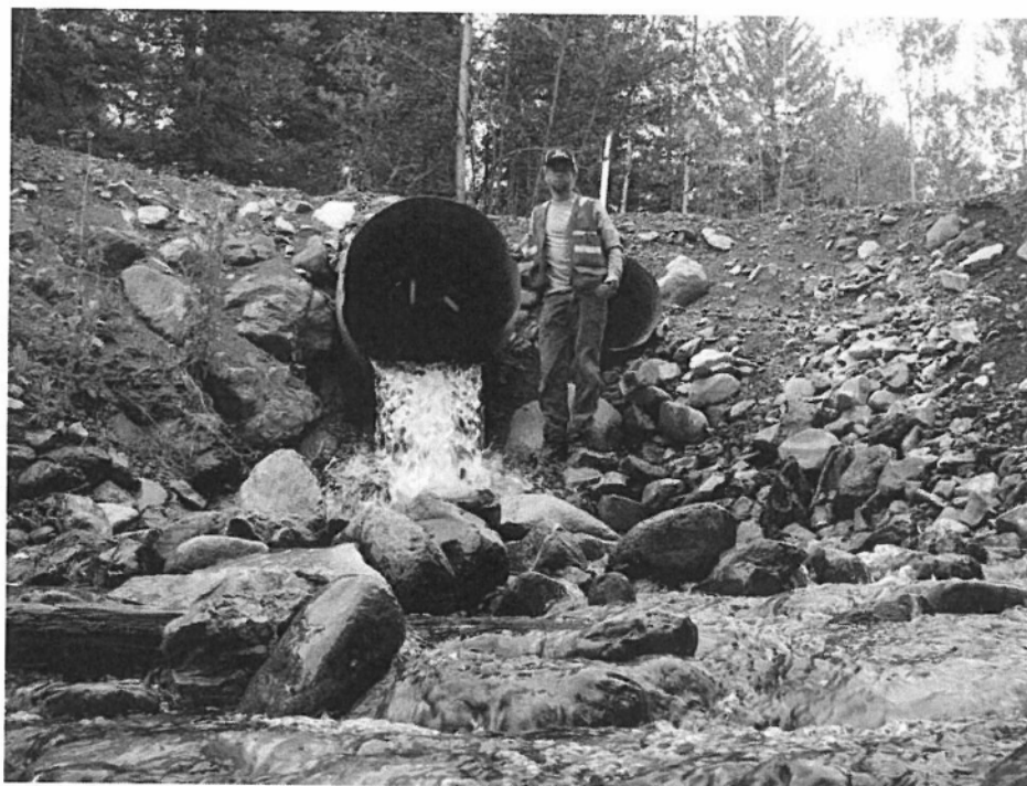
Photo 6: View of hanging culvert at Jim Creek crossing, 20 August 2007.
