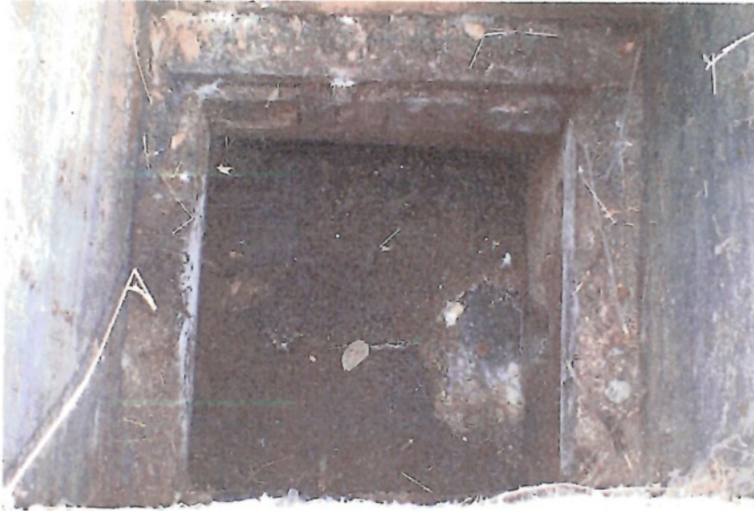
Photo 15 – Septic tank with lid removed (WP 15)
