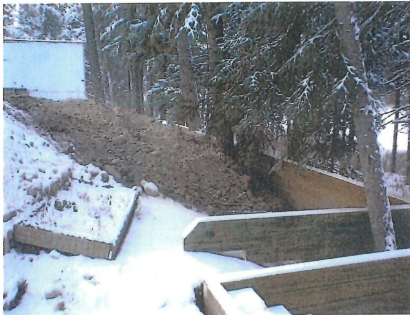
Photo 5 – Gravel, cobbles and coarse sand behind wooden retaining wall (WP 30)
