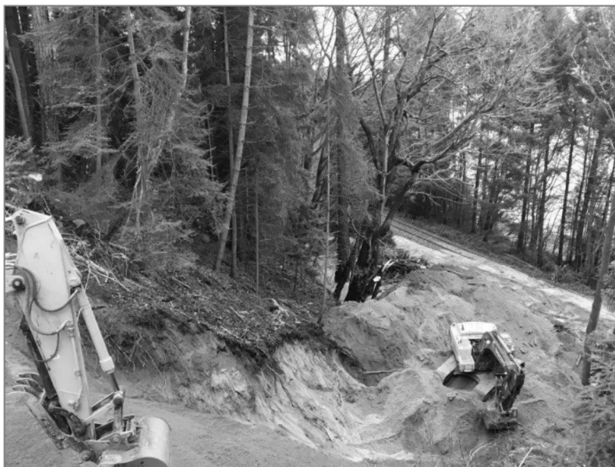
Photo 4: Looking down at the toe cleanup after sloughing of the western flank had occurred
