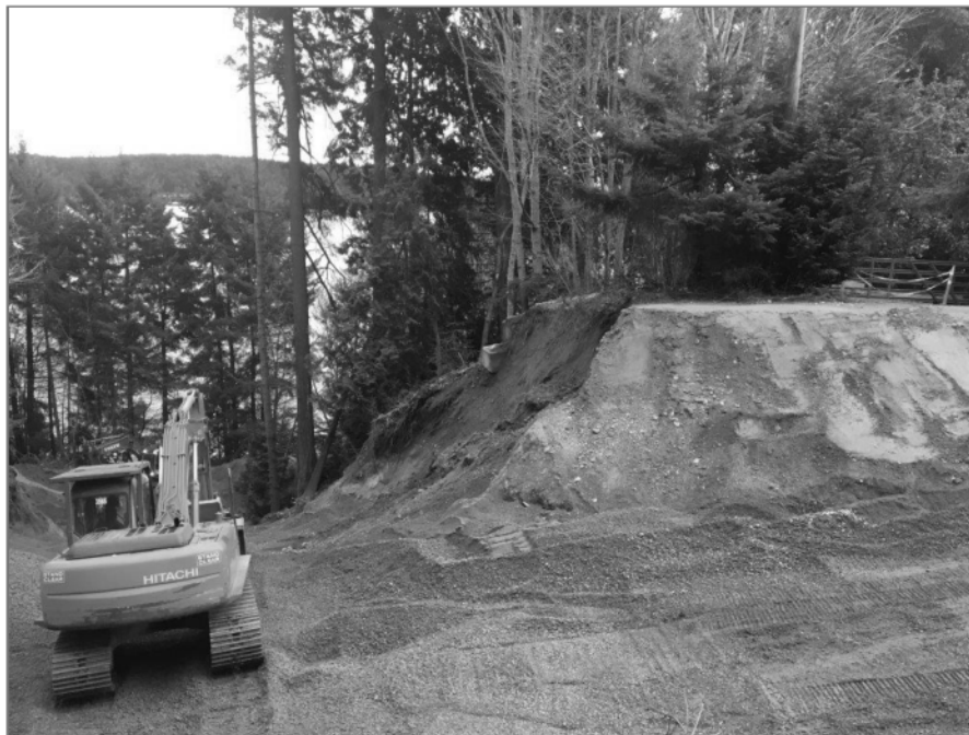
Photo 1: Sloughing on eastern shoulder of the failure sloughed into the work area. Approximately 1 m of horizontal ground was lost.
