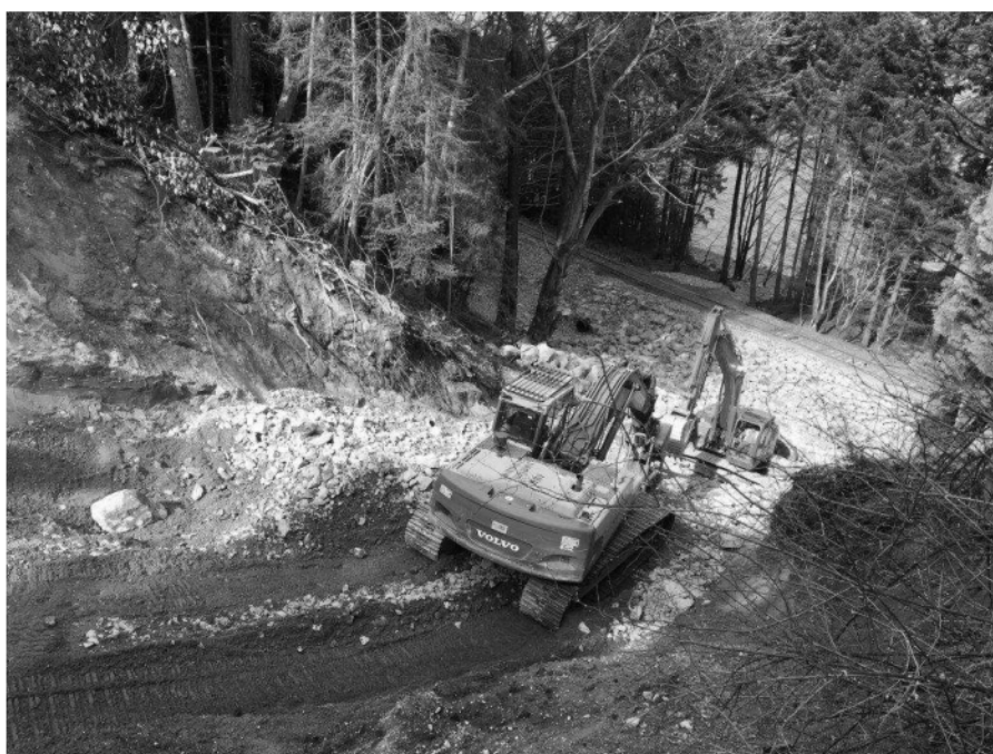
Photo 6: March 23, 2018. View looking downslope of the failure reconstruction progress. 18" Blast rock being mixed and track packed before graded to have swale surface.
