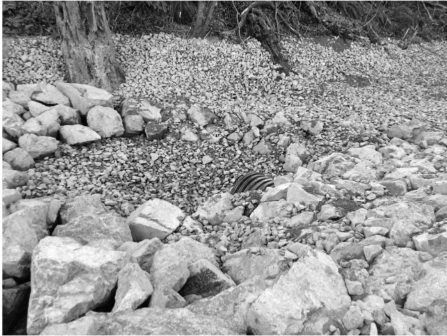
Photo 5: Complete collection pool at seaward outfall.
