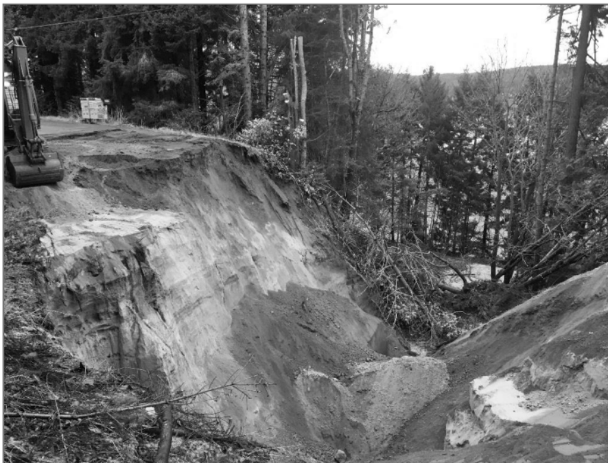
Photo 1: Excavator benching the gravel overburden on the west side of failure.
