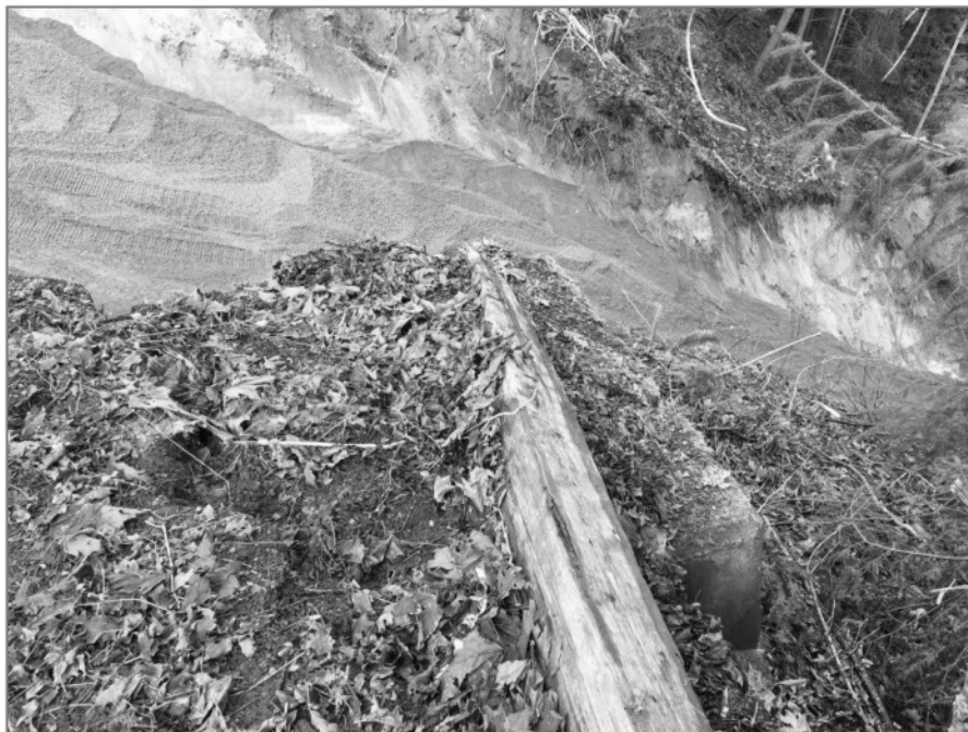
Photo 2: Tension crack behind lock block retaining wall on the east property.
