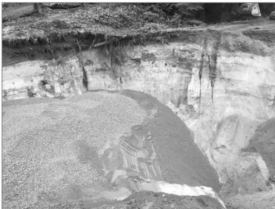
Photo 2: Filter sand being placed up sides of sand sidewalls on southern sidewall of failure.
