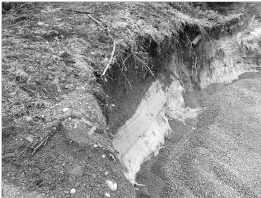
Photo 4: Sand filter material placed against southern (upstream) face of the failure. Generally greater than 0.6 m thick under the excess crush.
