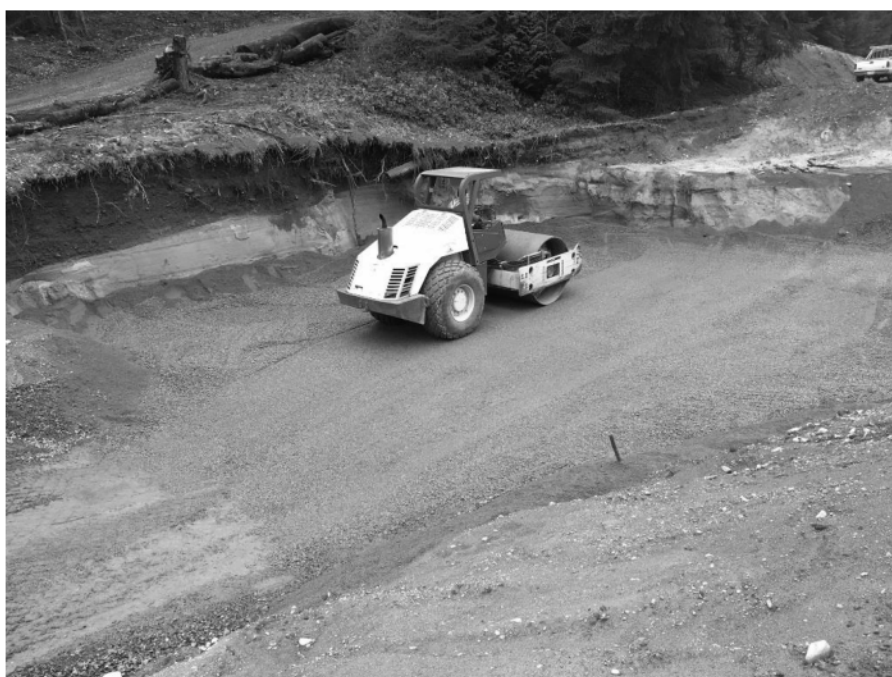
Photo 6: April 6, 2018. Packer at site to complete compaction of the road rebuild area. Lifts being placed at approximately 0.3 m.
