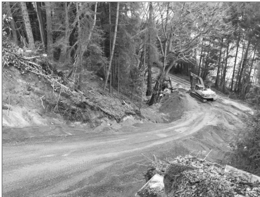
Photo 1: Continued progress on the removal of the waste material from the bottom of the failure.
