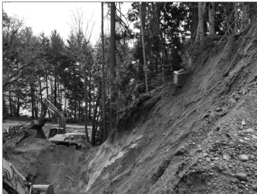
Photo 3: Lock blocks on east flank to be monitored and reviewed as part of the spotter's checks as the excavators work within the failure.
