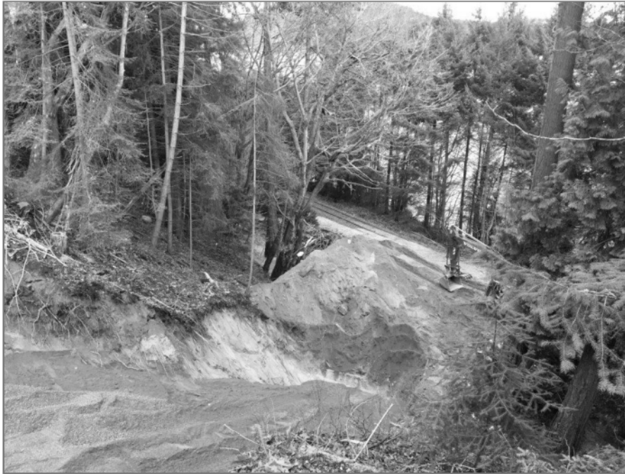
Photo 1: Excavator at toe continuing to stockpile loose material and clean out toe.
