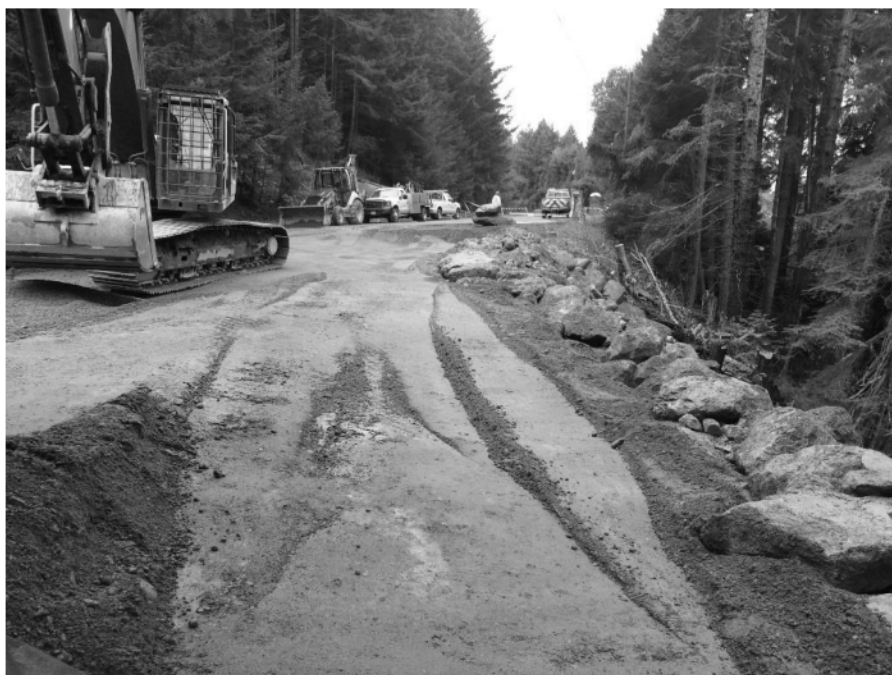
Photo 6: April 13, 2018. View looking west at the final slope reconstruction grade. Existing granular fill being spread out to level out area and transition the new construction with existing grades.
