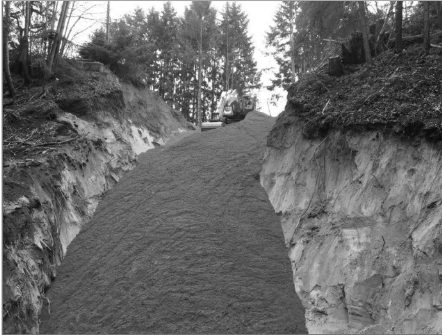
Photo 5: Sand being moved down the failure to cover the cleaned up toe excavations and help shore up the recent sloughing.
