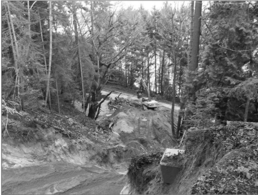
Photo 1: Excavator at toe continuing to stockpile loose material and sort wood debris, asphalt and sand.
