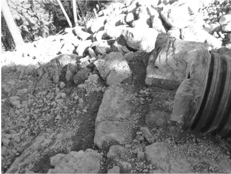
Photo 3: April 9, 2018. Culvert outfall area. Flat tabular particles placed to receive initial water discharge and dissipate water energy.
