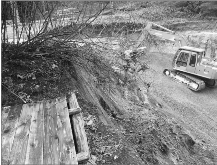
Photo 5: Sloughing that occurred in the morning. ~ 1 m lost on the western side of the hydro pole.
