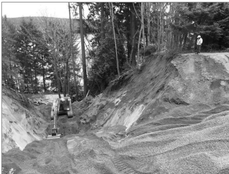
Photo 2: Excavator just over halfway down the slope, continuing to excavate loose material and asphalt debris.
