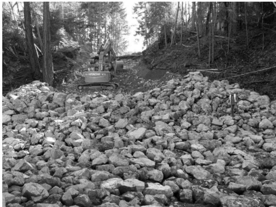
Photo 4: March 22, 2018. Looking upslope at riprap placement progress.
