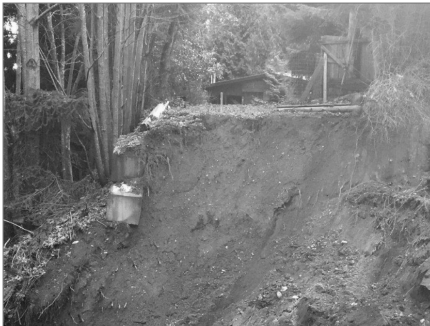
Photo 4: Fill material behind retaining wall obvious in section. Sloughing that occurred shown in right of image.
