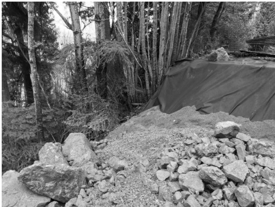
Photo 5: April 6, 2018. Area near the wooden retaining wall that requires some back sloping to provide base for tabular rocks to build up area.
