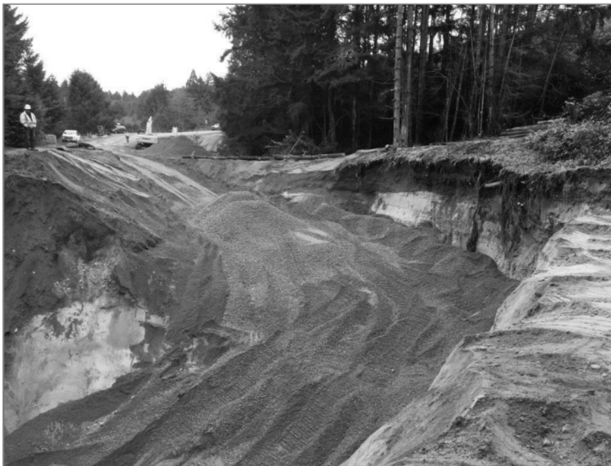
Photo 1: Progress of the ramp and access to the toe of the failure.
