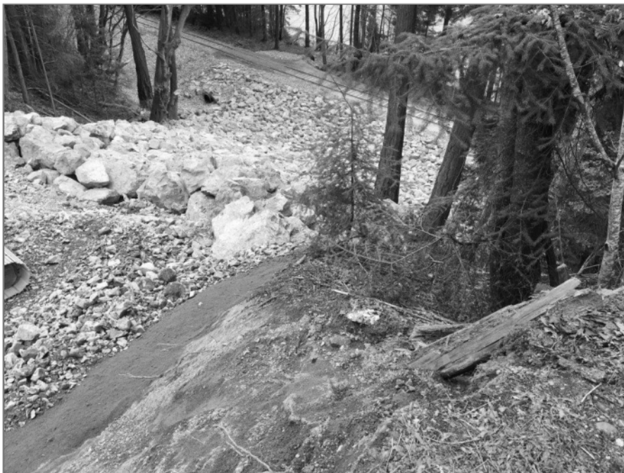
Photo 1: April 3, 2018. Looking down slope riprap construction and the recently removed lock block wall area.
