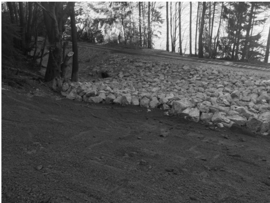
Photo 6: Completed riprap along base. Next step is importing and placing blast rock fill as the construction moves up the slope.
