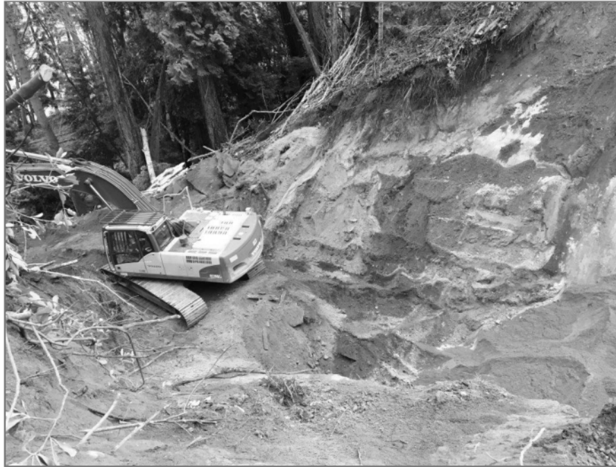
Photo 4: Excavation of loose material and asphalt to expose undisturbed subgrade reviewed, covered with sand filter. Progressed to over midway down slope.
