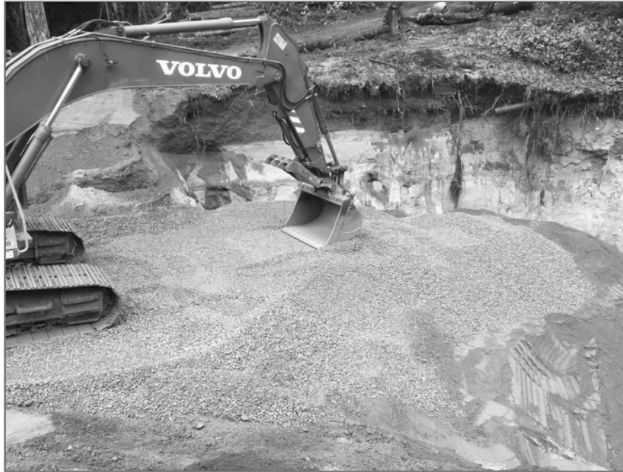
Photo 3: Crush travel surface being placed and tamped above sand filter.
