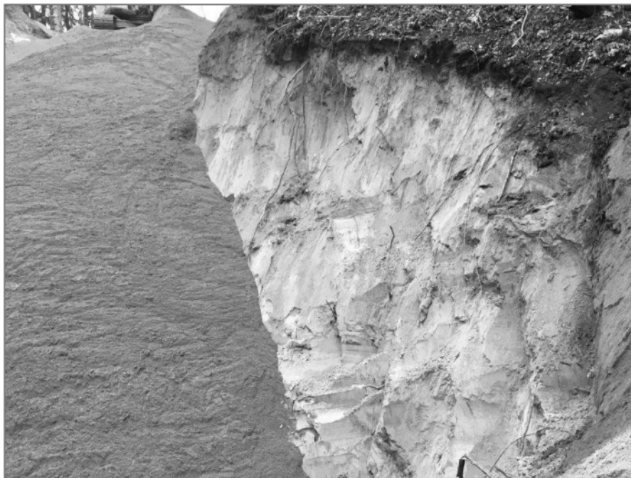
Photo 6: Cleaned up face of sloughed area.
