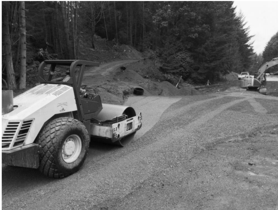
Photo 5: April 11, 2018. Placement and compaction of the pavement structure – Rumming Road.
