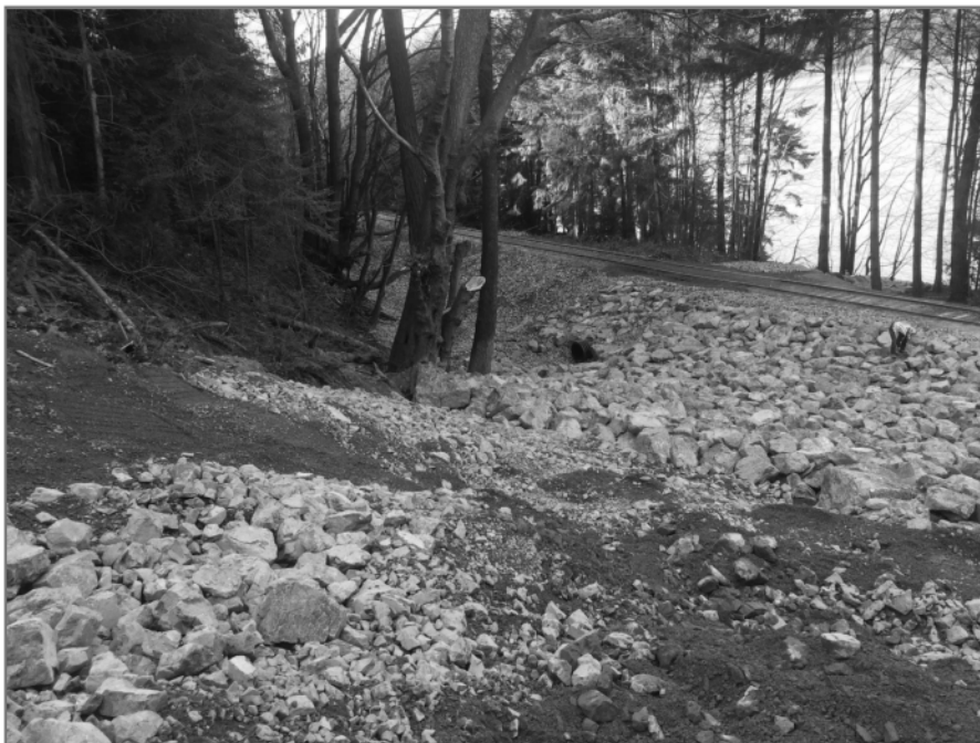
Photo 1: March 19, 2018. Looking down slope at the 18" blast rock placed
