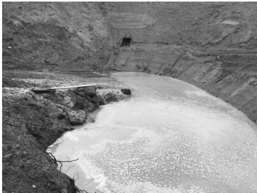
Photo 4: April 10, 2018. Sump area collecting stormwater from catchment areas. Contractor to monitor and reduce level as appropriate.
