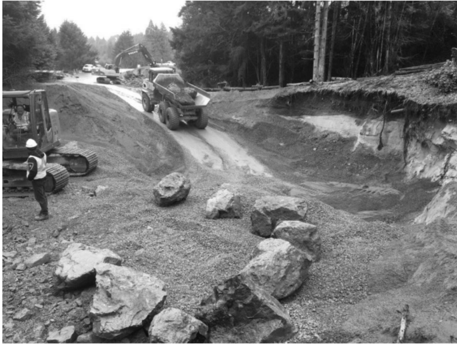
Photo 3: April 5, 2018. 1.5" crush hauled in to build up grades within the road prism.
