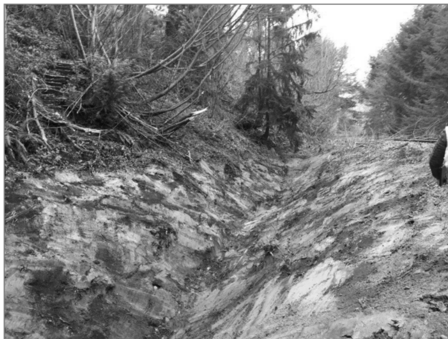
Photo 2: Cleaned out ditch towards the west from the bottom of the failure. Bottom of ditch appears ~3.5 m deep from top of railway.
