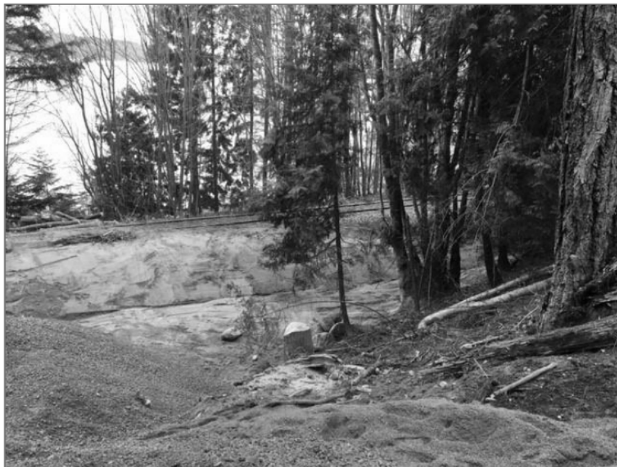
Photo 1: Looking down slope of the area that will require additional excavation to shore up upper areas of the slope. Stump to be removed and tree shown on right may need to be removed, however reconstruction will try work around.
