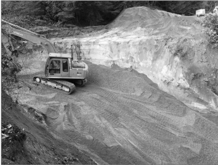
Photo 3: Contractor continuing to build up sand filter and crush material to help support existing sidewalls.
