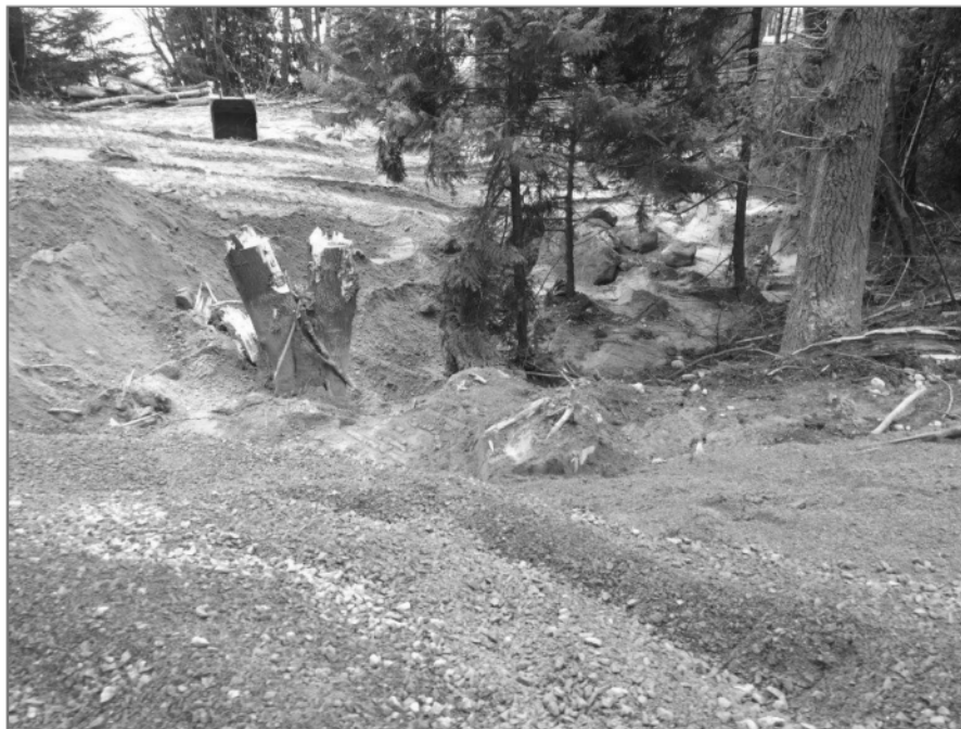
Photo 1: Looking down slope of the area that will require additional excavation to shore up upper areas of the slope. Stump to be removed and tree shown on right will likely be removed.
