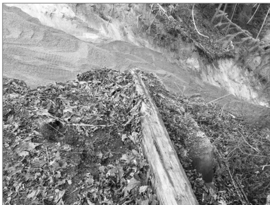
Photo 2: Tension crack behind lock block retaining wall on the east property.
