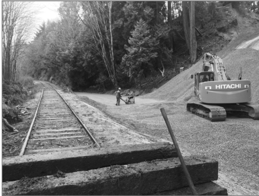
Photo 1: Looking east along the base of the slope at crush being placed and compacted.
