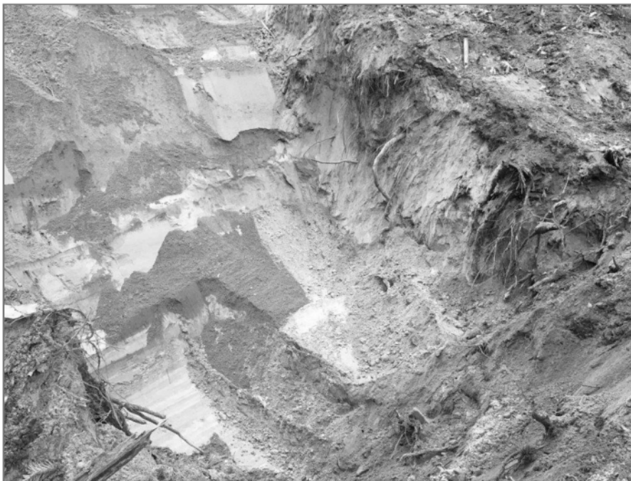
Photo 3: Excavations at the toe steepening due to depth of excavations to find undisturbed ground
