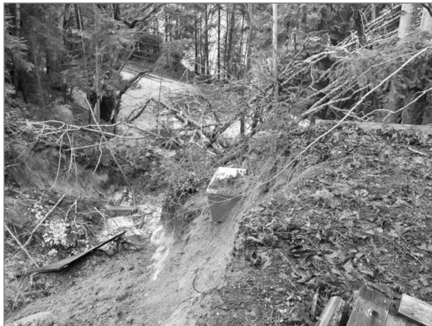
Photo 4: Several lock blocks had dislodged over the weekend and fallen into the failure. Several blocks remain and have distorted from original place. Tension crack visible behind the blocks.
