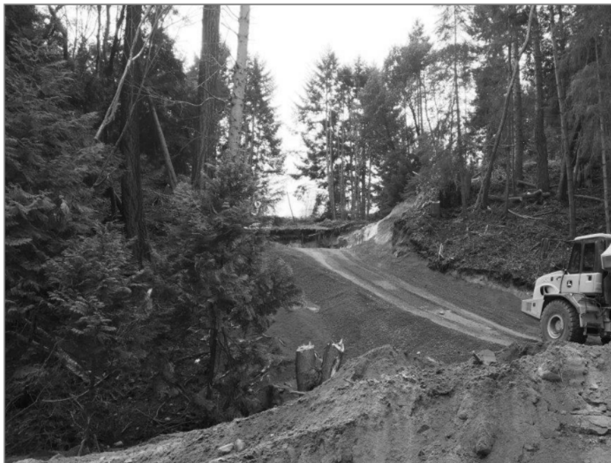
Photo 4: View looking up the failure. Some additional work to clean out the eastern toe will be required to help buttress the slope.
