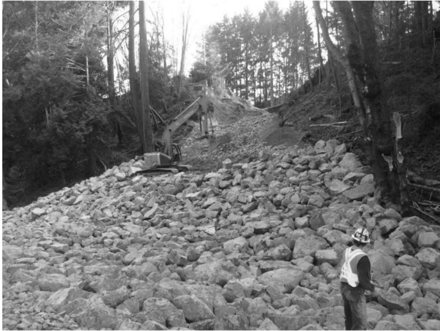
Photo 3: March 21, 2018. View looking upslope at the progress. Slope appears slightly overbuilt from designed slope. Field fit adjustments and ease of track packing contributing to overbuilt.
