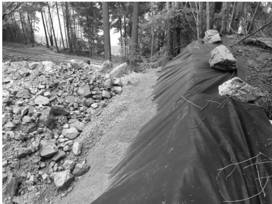
Photo 4: April 5, 2018. Geotextile place along eastern property cut and retaining wall area.
