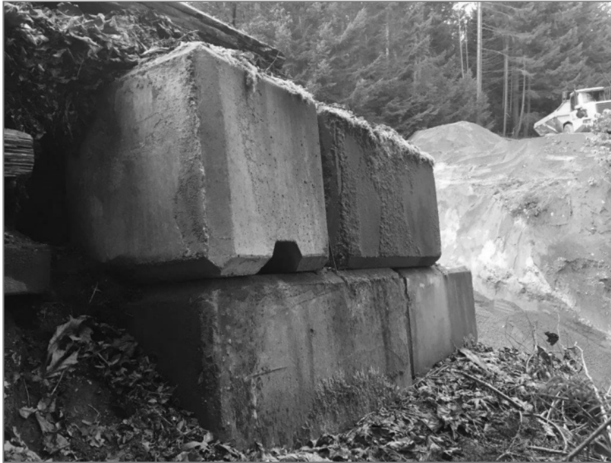
Photo 3: Lock block retaining wall on eastern property.
