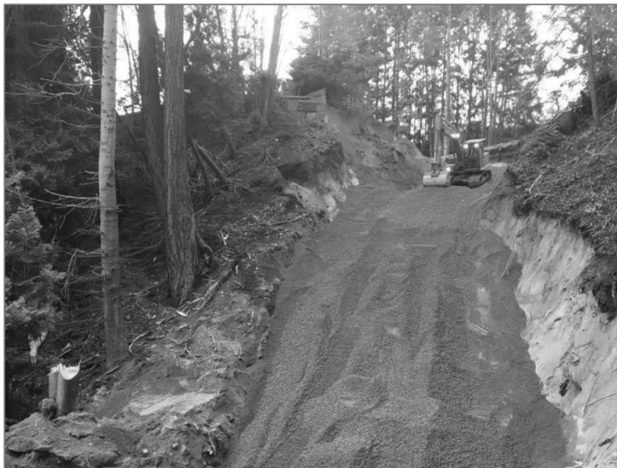
Photo 6: Progress of the access road down to the toe of failure.
