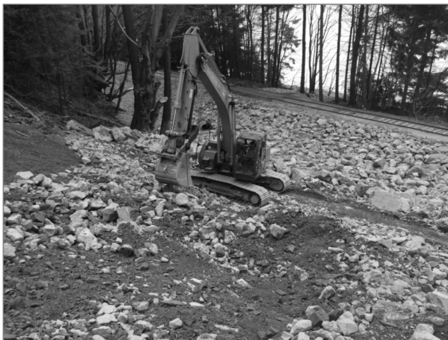
Photo 2: March 20, Excavator track packing the 18" blast rock material.
