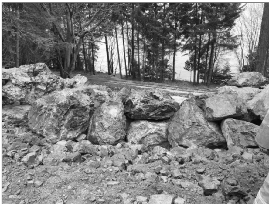
Photo 2: April 4, 2018, Swale being developed in the riprap subsequent granular layers.
