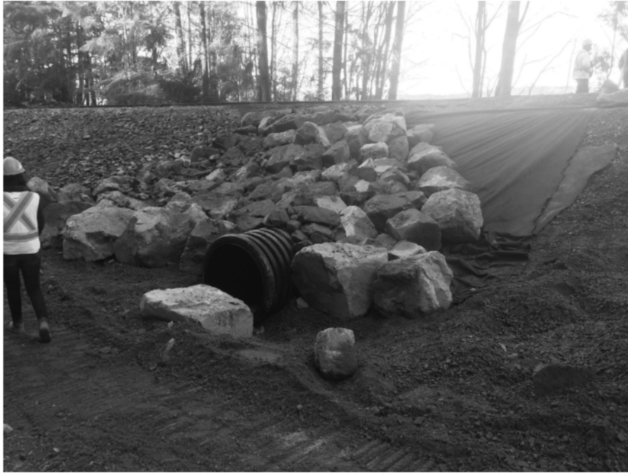
Photo 3: Inlet side of seaward outfall.
