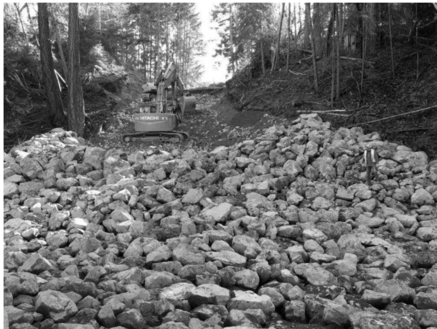
Photo 4: March 22, 2018. Looking upslope at riprap placement progress.
