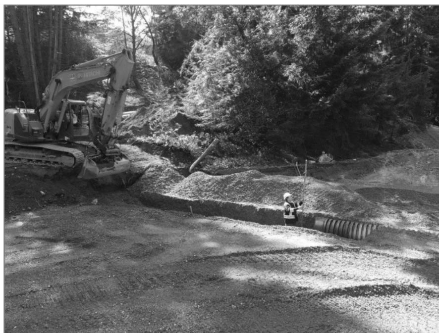
Photo 2: April 10, 2018. Culvert being placed in the Rumming Road reconstruction.
