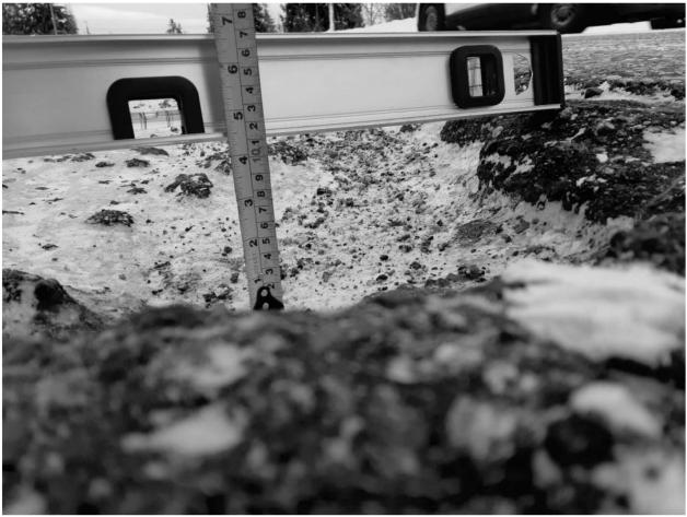
The pothole above is on the Northbound Travelled Lane of Hwy 97B and is over 100mm deep.
