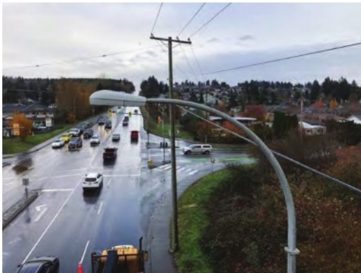
Investigate clearances at adjacent pole due to removal of 8 m pole with updated 8.5 m pole replacement
