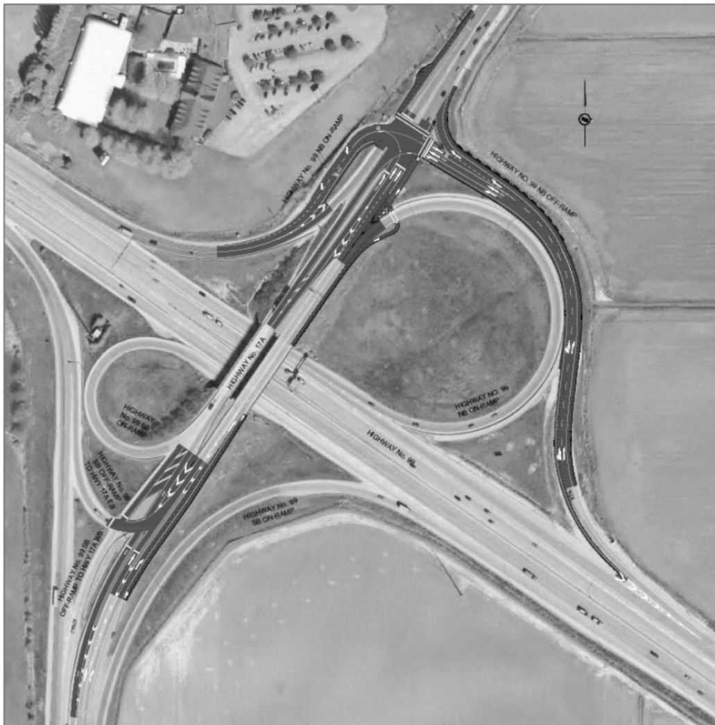
Figure 10: Highway 99 and 17A Off-Ramp Widening
