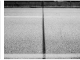
Filename: 018 02840E pier 2 compression seal joint.JPG
