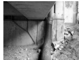
Filename: 090 02840W south abutment west end large delam in the breastwall at the drain.JPG
