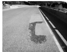
Filename: 013 02836E span 3 slow lane asphalt filled pothole.JPG
