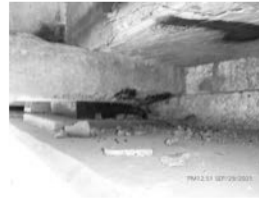
Filename: 078 02840W pier 2 south face spall and exposed rebar in the bottom flange of girder 3D.JPG
