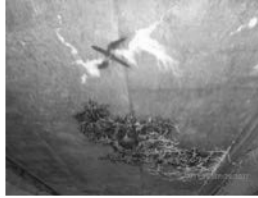
Filename: 044 02840W span 1 bay 2 at the north abutment cracks and efflorescence in the subdeck.JPG
