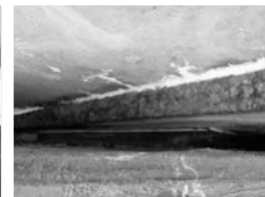
Filename: 042 02836E pier 2 span 3 bearing C elastomeric with Teflon and stainless.JPG
