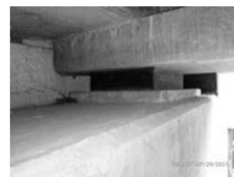
Filename: 052 02840E pier 2 span 3 laminated elastomeric bearings.JPG
