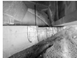
Filename: 053 02836W south abutment large delams in the breastwall between girders D and E.JPG
