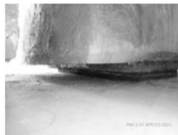
Filename: 032 02836E pier 1 span 2 bearing A elastomeric bearing with Teflon and stainless cracks pad.JPG
