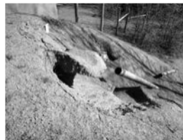
Filename: 005 02836E south east corner drain pipe disconnected and fill washed out.JPG
