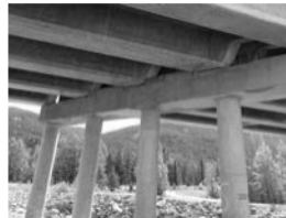
Filename: 2015 spall other side of column. this photo shows cap delam.JPG
