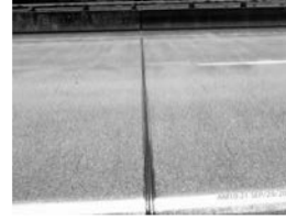
Filename: 016 02840W pier 1 compression seal joint.JPG
