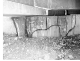
Filename: 025 02836W north abutment west end large delam in the breastwall under girder E.JPG
