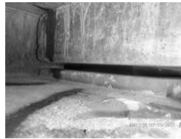
Filename: 041 02840W north abutment typical plain elastomeric bearings.JPG
