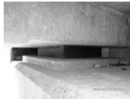
Filename: 074 02840W pier 2 span 3 laminated elastomeric bearings.JPG
