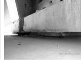
Filename: 037 02836W pier 2 bearing D elastomeric with Teflon and stainless.JPG
