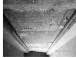
Filename: 045 02836E span 3 bay 3 efflorescence and delams in the subdeck.JPG
