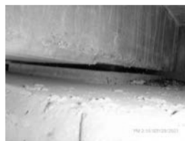
Filename: 045 02840E pier 1 span 2 plain elastomeric bearings.JPG
