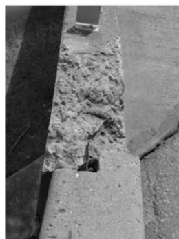
Filename: 2012 parapet defect.JPG
