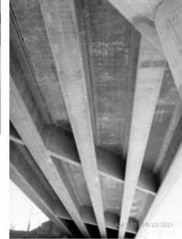
Filename: 044 02836E span 3 looking north eff and cracking in bay 4 at pier 2.JPG
