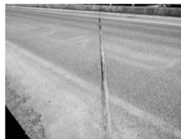
Filename: 007 02836W pier 1 compression seal joint.JPG
