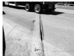
Filename: 014 02836W south abutment compression seal joint falling through.JPG
