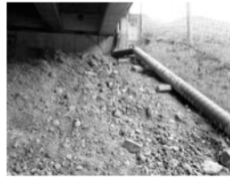
Filename: 091 02840W south abutment west end embankment scour along the drain pipe.JPG
