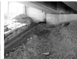
Filename: 027 02836E south abutment east end embankment scour exposing the footing.JPG
