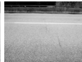
Filename: 017 02840E span 2 transverse cracks in the wearing surface.JPG
