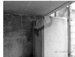
Filename: 040 02840W north abutment east end delam in the shear key.JPG
