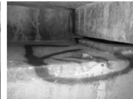
Filename: 045 02840W north abutment bay 4 small delam in the top of the bearing area.JPG
