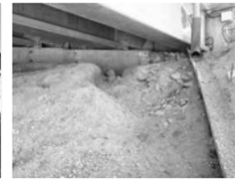
Filename: 048 02836W south abutment west end embankment scour.JPG
