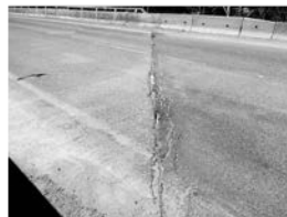
Filename: 003 02836W north abutment no joint.JPG
