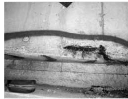
Filename: 077 02840W pier 2 south face bay 3 large delam in the bottom of the diaphragm.JPG
