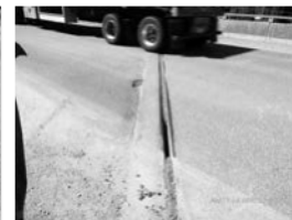
Filename: 014 02836W south abutment compression seal joint falling through.JPG
