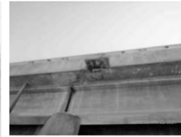
Filename: 035 02836W span 2 pier 2 west end large spall with exposed rebar underside of the luminaire.JPG
