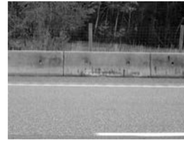
Filename: 005 02840W north approach west side delams and spalls in the approach flare.JPG
