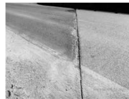
Filename: 016(02836E)2021 north abutment no joint.JPG
