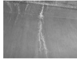
Filename: 043 02836W span 3 girder C eff and fine vertical crack in the web of the girder.JPG
