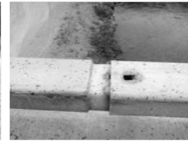
Filename: 019 02840E pier 2 east side missing connection bolt in the parapet railing.JPG
