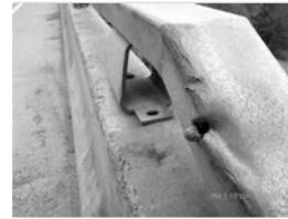
Filename: 012 02480E south abutment east end of the rail impact damage and missing bolt.JPG
