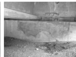
Filename: 064 02840E north abutment bay 4 delamination in diaphragm.JPG
