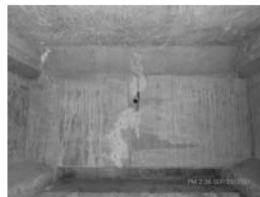
Filename: 063 02840E north abutment bay 2 horizontal seismic restraint bolt is missing.JPG
