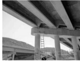
Filename: 029 02836W pier 1 north face east end medium delam in the top corner.JPG
