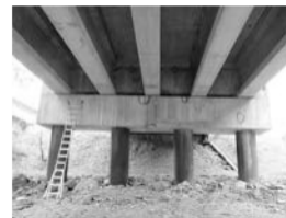
Filename: 065 02840W pier 2 north face small delams in the cap.JPG
