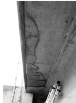
Filename: 053 02840W span 1 west side delams in the soffit.JPG
