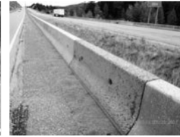
Filename: 006 02840W north approach east flare 1 CRB with small spalls.JPG
