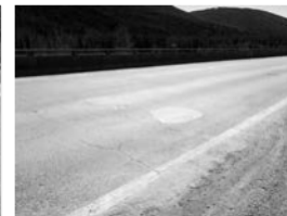
Filename: 005 02836W span 1 slow lane cracks and patches in the wearing surface.JPG
