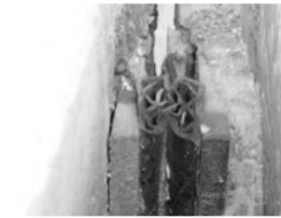
Filename: 020 02840W pier 2 end of the compression seal joint.JPG
