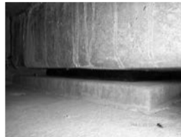
Filename: 034 02840E south abutment typical plain elastomeric bearing.JPG
