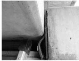
Filename: 059 02840W pier 1 span 1 west end wear plate corroding.JPG
