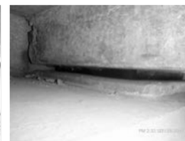
Filename: 061 02840E north abutment plain elastomeric bearing.JPG
