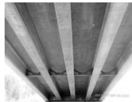
Filename: 052 02840 span 1 steel diaphragms .JPG
