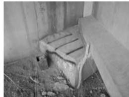
Filename: 051 02836E north abutment west end delam in the bearing seat.JPG
