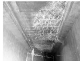
Filename: 028 02836W north abutment span 1 bay 4 cracking and heavy eff in the subdeck.JPG
