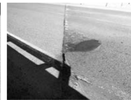
Filename: 017(02836E)2021 north abutment east side large pothole in the approach.JPG
