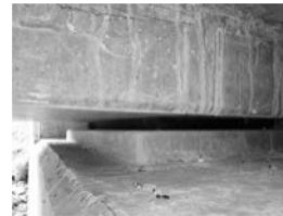
Filename: 083 02840W south abutment typical plain elastomeric bearings.JPG
