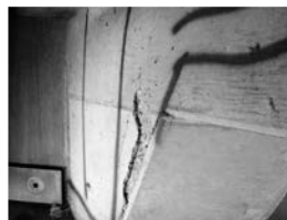
Filename: 038 02836W pier 2 span 3 bay 4 large delam in the diaphragm.JPG
