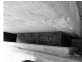
Filename: 058 02840W pier 1 span 1 laminated elastomeric bearings.JPG
