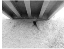
Filename: 059 02840E north abutment embankment scour.JPG
