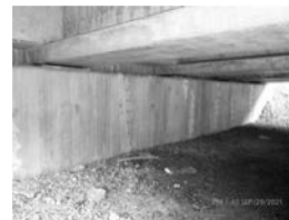
Filename: 035 02840E south abutment epoxy injection ports in the breast wall.JPG
