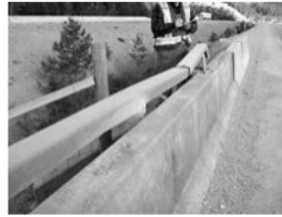
Filename: 014 02836E north west corner damage to the parapet railing.JPG
