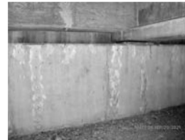
Filename: 039 02840W north abutment numerous epoxy sealed vertical cracks in the breastwall.JPG
