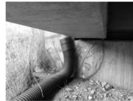
Filename: 037 02840E south abutment east end delam at the drain pipe.JPG
