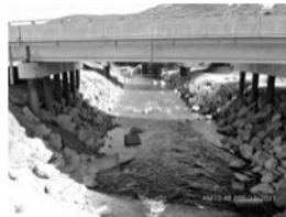
Filename: 018 06006 rip rap on the downstream channel looking east.JPG
