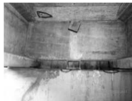
Filename: 047 02840W north abutment horizontal and vertical seismic restraints in the outside bays.JPG
