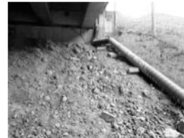
Filename: 091 02840W south abutment west end embankment scour along the drain pipe.JPG
