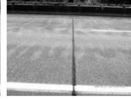
Filename: 019 02840W pier 2 compression seal joint.JPG
