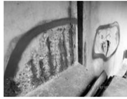
Filename: 043 02840E pier 1 east end delams, spalls and exposed rebar in the webs of girders 1E and 2E.JPG
