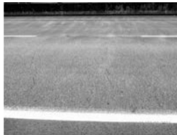
Filename: 014 02840W span 1 transverse cracks in the wearing surface.JPG
