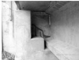
Filename: 049 02840W north abutment west end delam in the ballast wall.JPG
