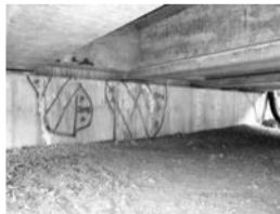
Filename: 085 02840W south abutment large delams in the breast wall between girders B and C.JPG
