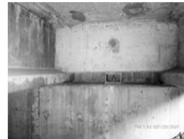
Filename: 036 02840E south abutment bay 1 vertical seismic restraint but no horizontal.JPG
