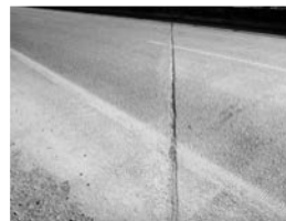
Filename: 010 02836E pier 1 compression seal joint.JPG
