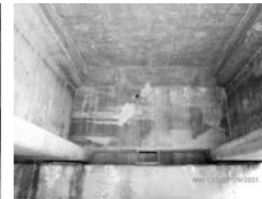
Filename: 042 02840W north abutment bay 1 missing horizontal seismic restraint.JPG
