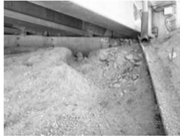
Filename: 048 02836W south abutment west end embankment scour.JPG
