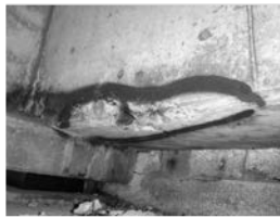
Filename: 075 02840W pier 2 south face bay 2 delam and spall in the bottom of the diaphragm.JPG
