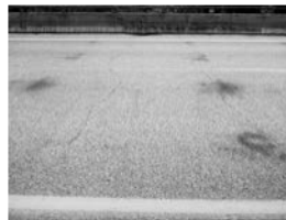
Filename: 014 02840E span 1 transverse cracks in the wearing surface.JPG
