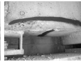
Filename: 079 02840W pier 2 south side bay 4 delam in the diaphragm.JPG
