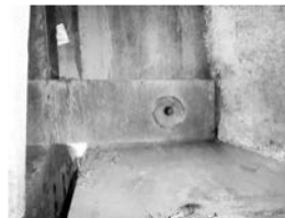
Filename: 039 02836W pier 2 girder D connection plated bolt broken on the east side.JPG
