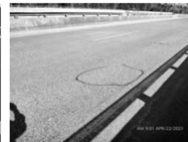
Filename: 009 02836E span 1 delams in the wearing surface.JPG
