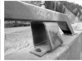
Filename: 012 02840W north abutment west parapet rail first rail post pedestal is cracked.JPG
