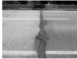
Filename: 009 02840E south abutment no joint.JPG
