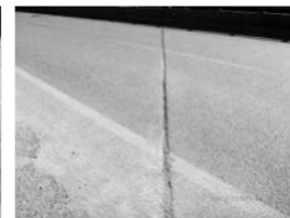
Filename: 012 02836E pier 2 compression seal joint.JPG
