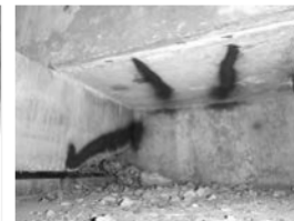
Filename: 070 02840W pier 2 north side delam in the underside of the diaphragm in bay 3.JPG
