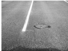
Filename: 010 02840W span 1 small pothole near the north abutment.JPG
