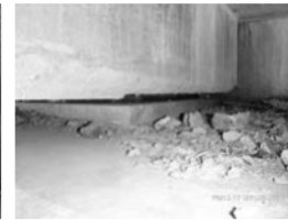
Filename: 069 02840W pier 2 span 2 plain elastomeric bearing.JPG
