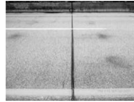
Filename: 015 02840E pier 1 compression seal joint.JPG
