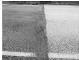
Filename: 023 02840E north abutment no joint.JPG
