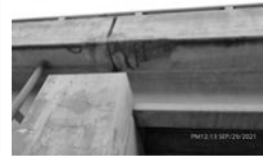
Filename: 066 02840W pier 2 west end delams in the soffit at the joint.JPG
