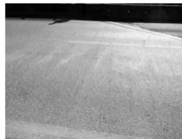
Filename: 008 02836E span 1 extensive cracking in the wearing surface.JPG
