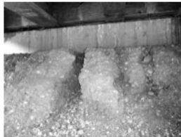
Filename: 037 02840W north abutment embankment scour.JPG
