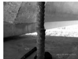
Filename: 041 02836E pier 2 seismic restraints broken and welded.JPG
