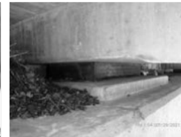
Filename: 042 02840E pier 1 span 1 laminated elastomeric bearing.JPG
