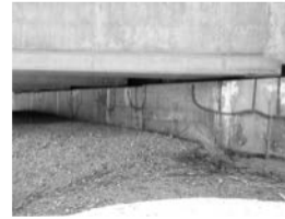
Filename: 029 02836E south abutment delams in the breastwall.JPG
