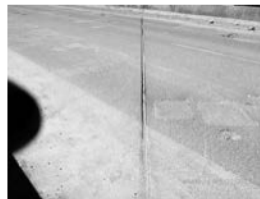
Filename: 009 02836W pier 2 compression seal joint.JPG
