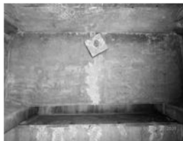
Filename: 043 02840W north abutment epoxy filled cracks in the concrete diaphragms.JPG
