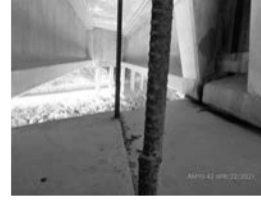
Filename: 032 02836W pier 1 vertical seismic restraints.JPG
