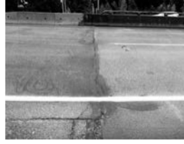
Filename: 008 02840W north abutment no joint.JPG
