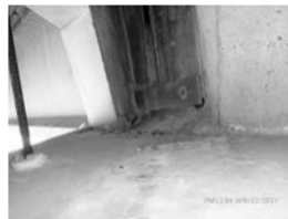
Filename: 034 02836E pier 1 girder D bottom flange connection plate bolt broken.JPG
