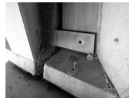
Filename: 040 02836W pier 2 girder E connection plate bolt broken.JPG
