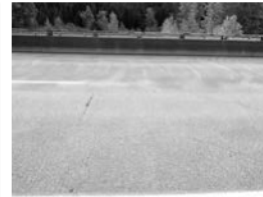
Filename: 018 02840W span 2 transverse cracks in the wearing surface.JPG
