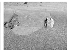
Filename: 010 02836W span 2 large deep pothole in the slow lane near pier 2.JPG
