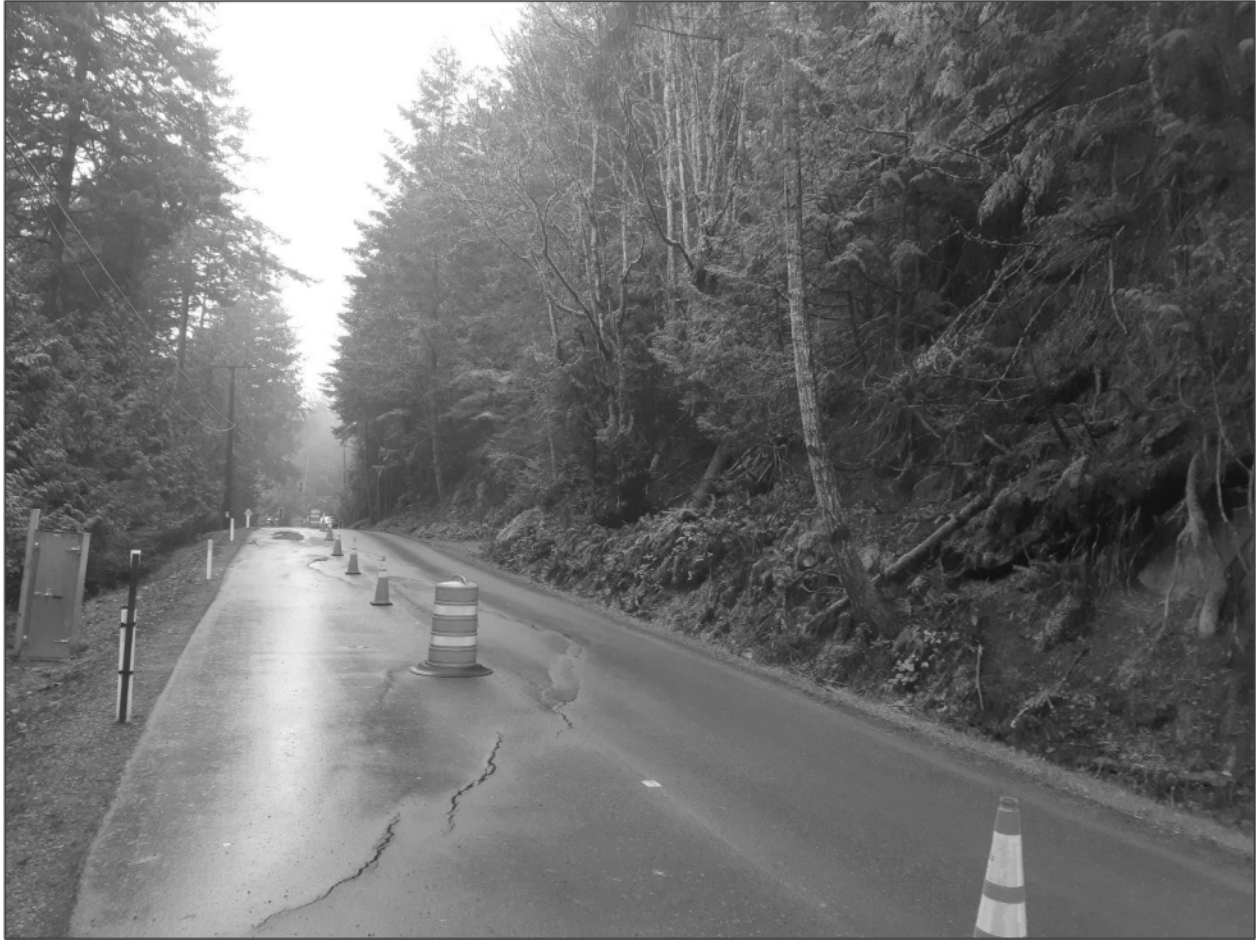
Figure 2. Canal Road on South Pender Island, BC - image of the longitudinal pavement crack and steep terrain above the road (view from the West to the East).
