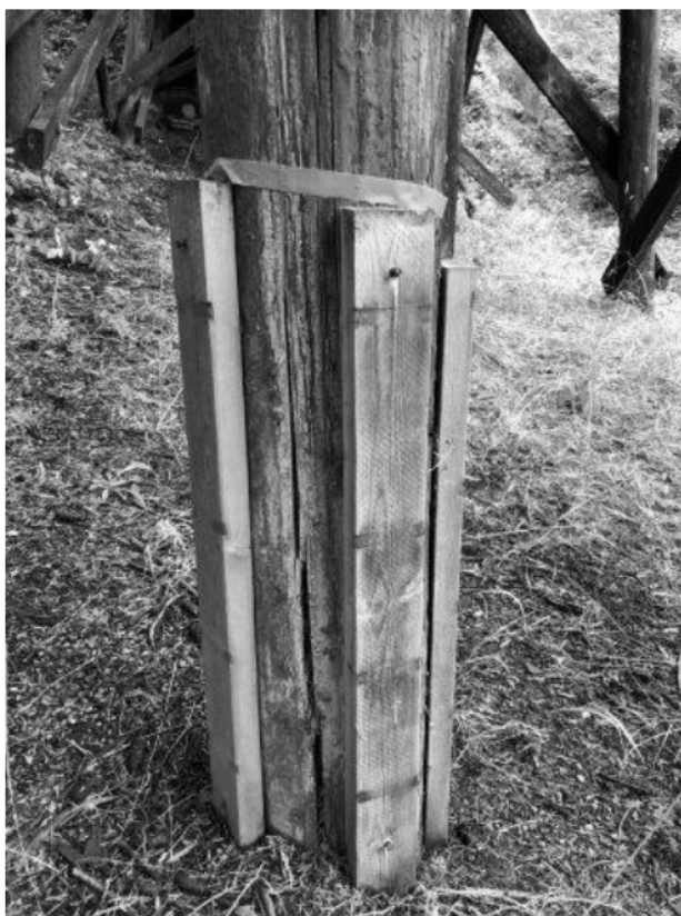
Photo 12 – Pier 4 Failed Pile Clamp Repair
