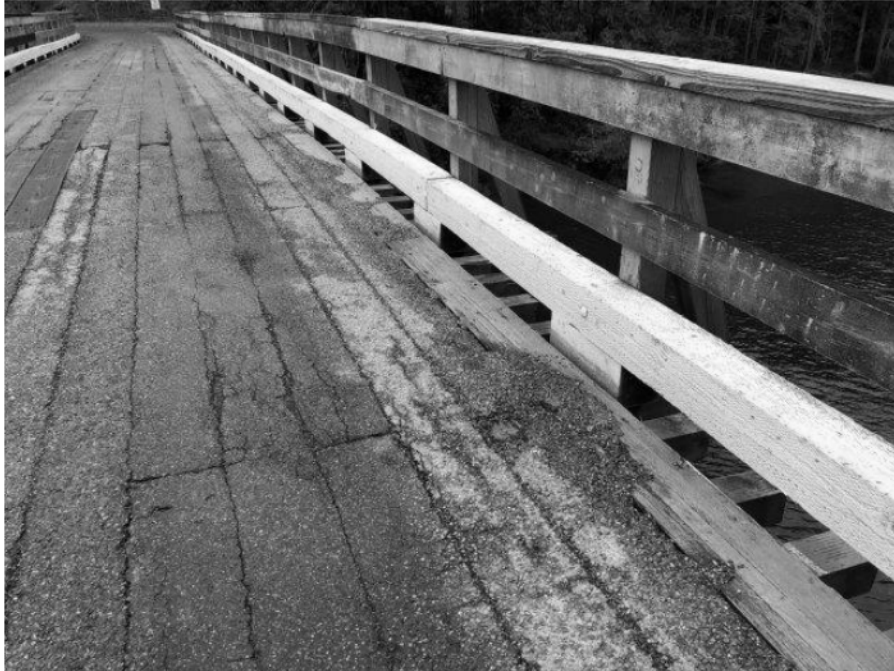
Photo 5 – Typical Condition of Timber Curb and Handrail
