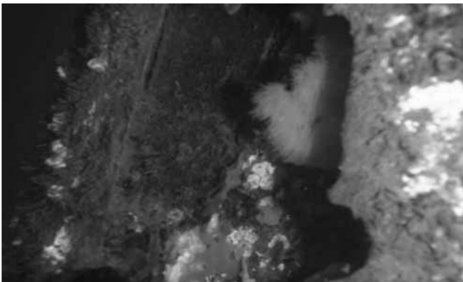
Photo 10: Canal Bridge No. 6880 - severe deterioration due to marine borer attack on Pile No. 4 on Pier No. 8.
