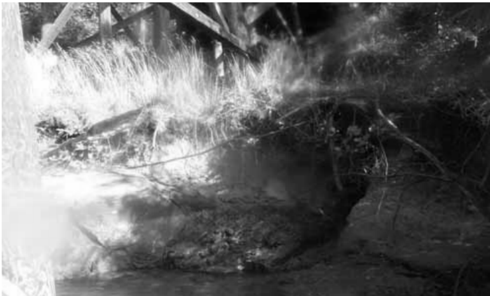
Photo 21: Canal Bridge No. 6880 - erosion of the embankment adjacent to Pier No. 4.
