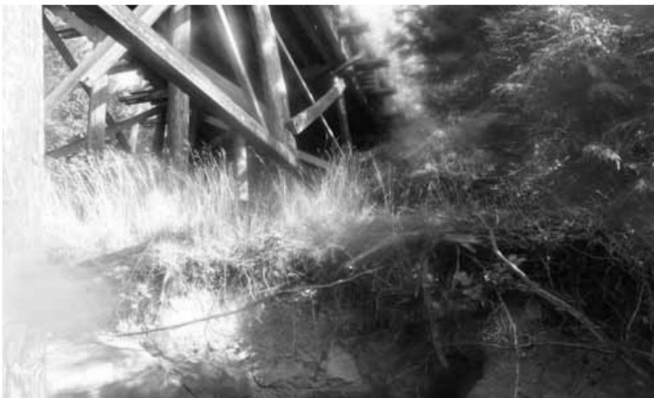
Photo 20: Canal Bridge No. 6880 - erosion of the embankment adjacent to Pier No. 4.
