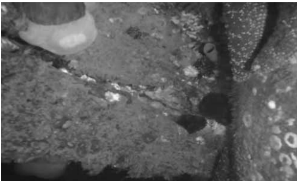
Photo 16: Canal Bridge No. 6880 - severe deterioration due to marine borer attack to a cross-brace on Pier No. 6.
