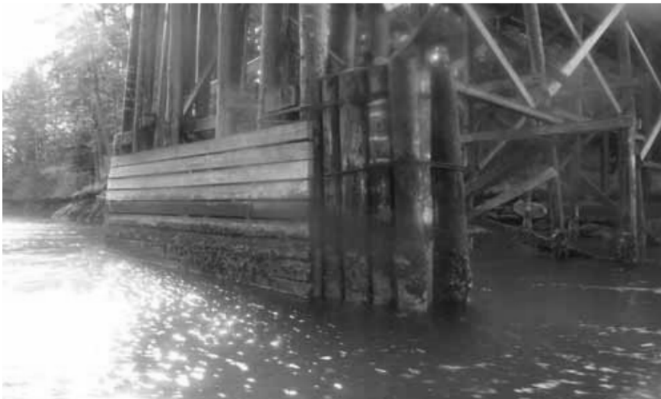
Photo 4: Canal Bridge No. 6880 - 7-pile fender group on the northwest side on Pier No. 8.
