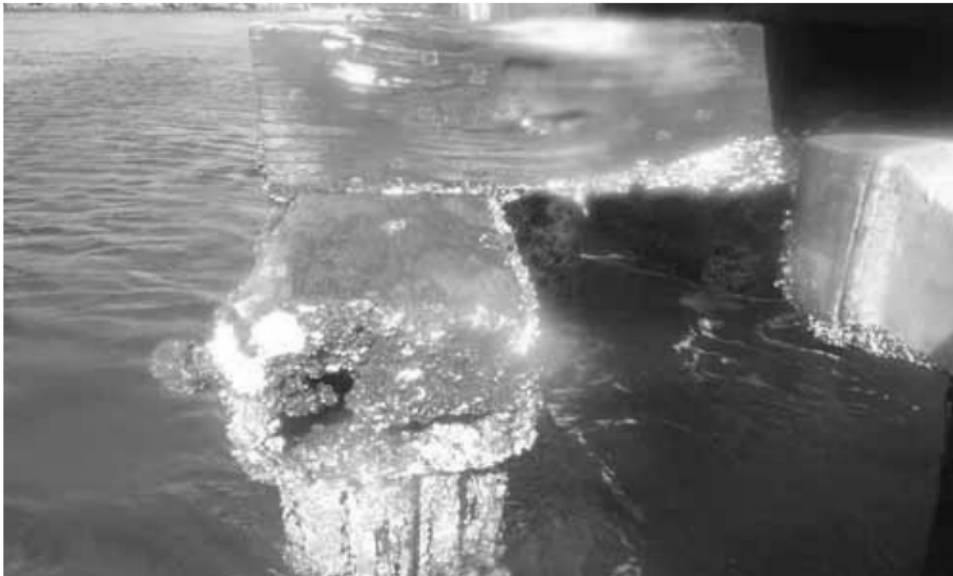
Photo 5: Canal Bridge No. 6880 - severe fungal decay to the southwest sub-cap on Pier No. 6.
