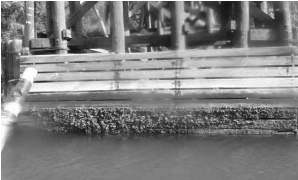
Photo 19: Canal Bridge No. 6880 - horizontal sheeting timbers on Pier No. 7.
