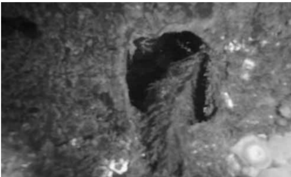
Photo 8: Canal Bridge No. 6880 - severe deterioration due to marine borer attack on Pile No. 9 on Pier No. 6.
