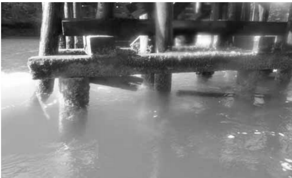
Photo 6: Canal Bridge No. 6880 - typical minor fungal decay to the pile caps on Pier No. 6.
