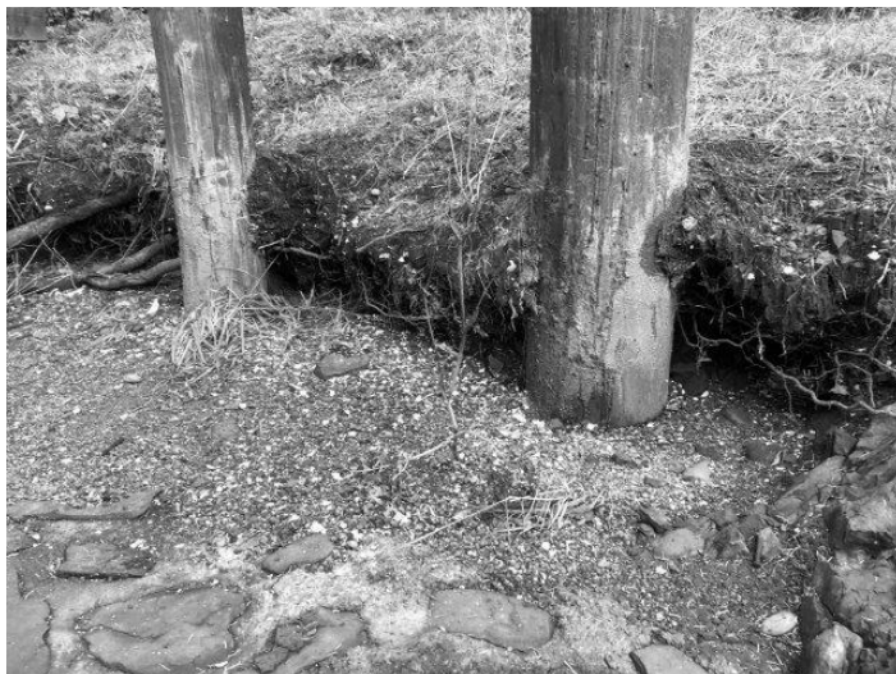
Photo 15 – Pier 5 Erosion at Base of Piles
