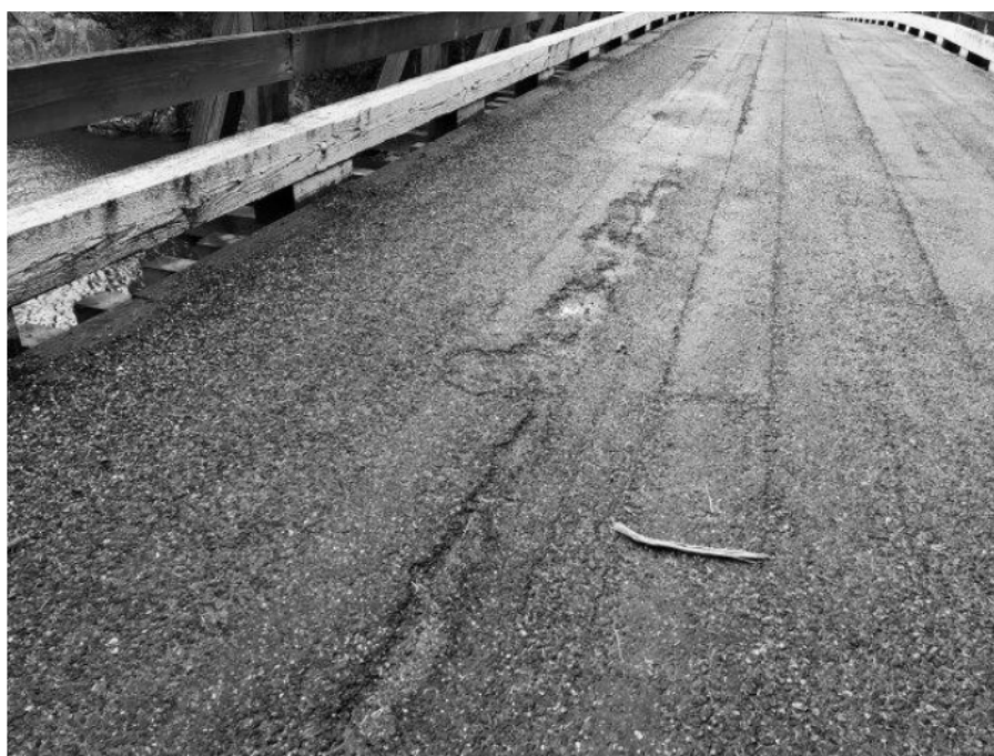
Photo 4 – Deterioration of Asphalt Wearing Surface
