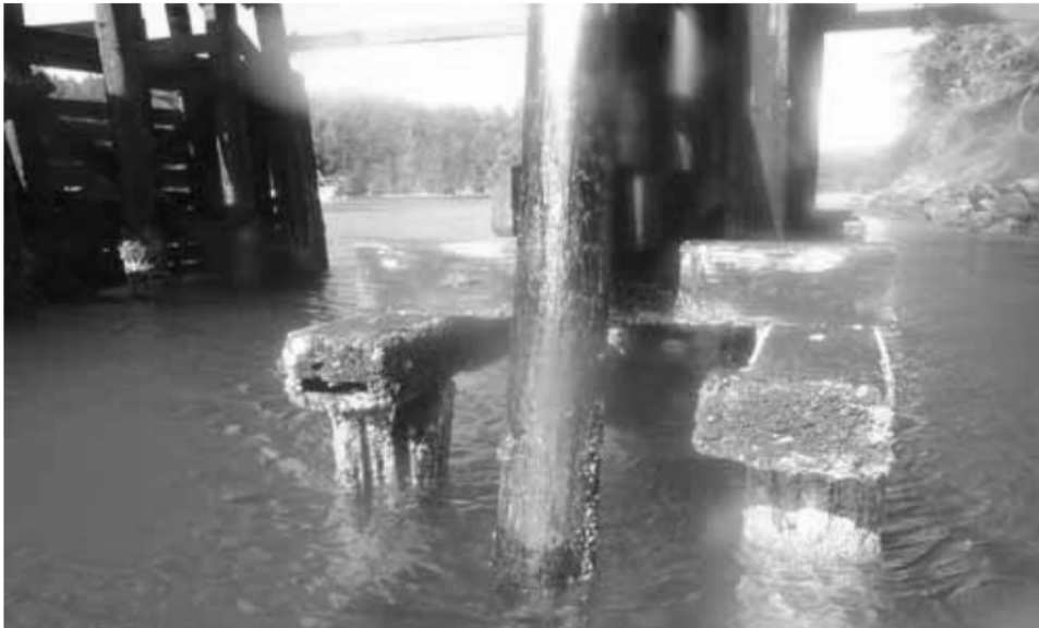
Photo 9: Canal Bridge No. 6880 - severe deterioration due to marine borer attack on Pile No. 13 on Pier No. 6.
