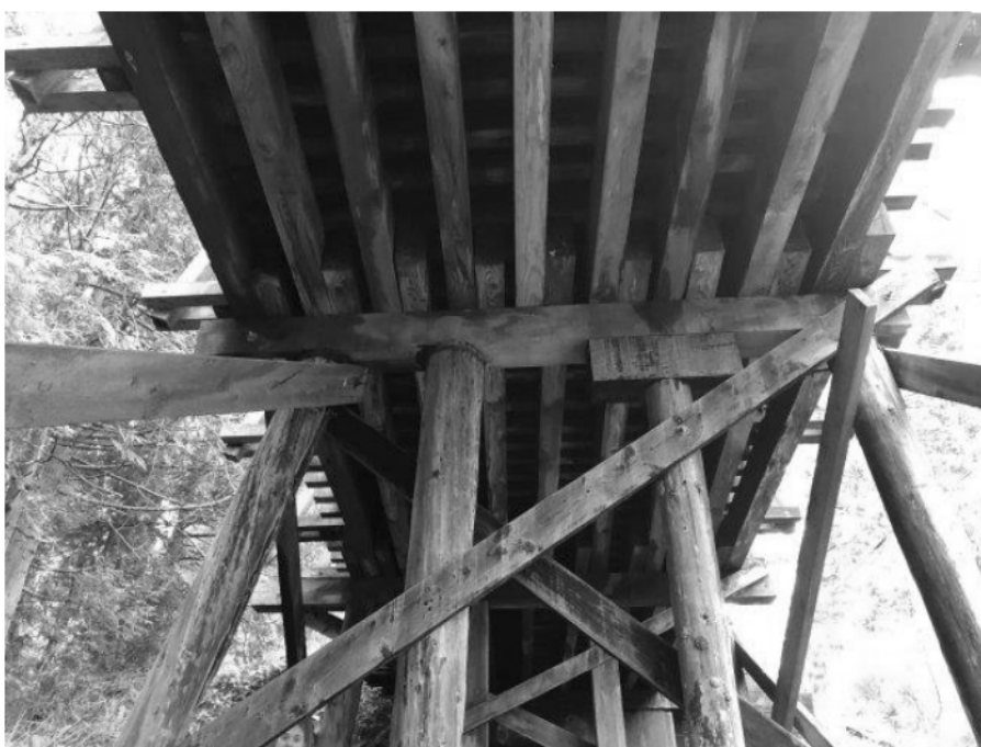
Photo 8 – Pier 2 Typical View (sub-cap installed under Pile B, second from east [right] side)
