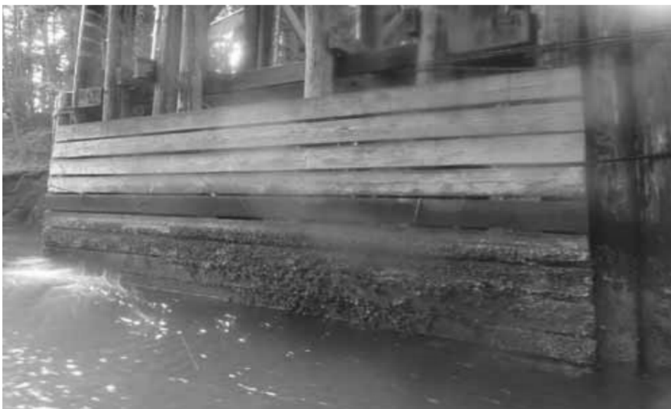
Photo 18: Canal Bridge No. 6880 - horizontal sheeting timbers on Pier No. 8.
