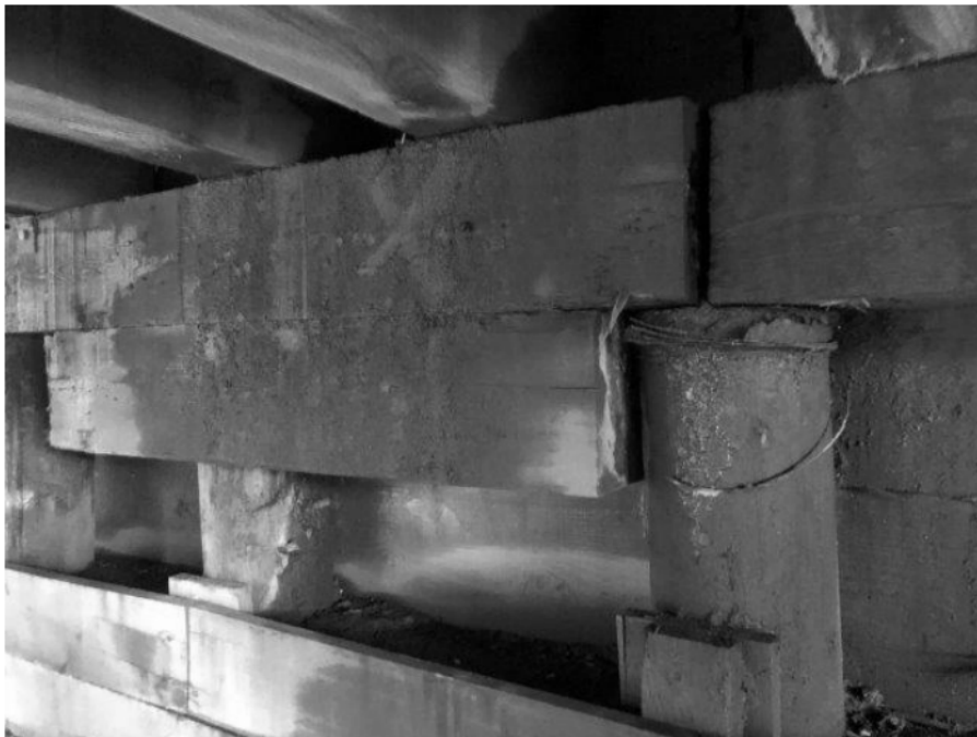
Photo 28 – Pile Cap and Corbel Block Inadequately Secured
