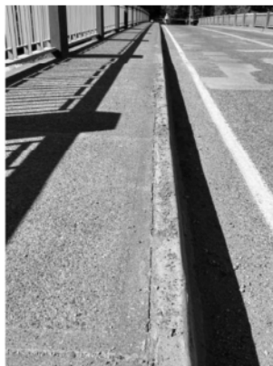
Sidewalk. Material in joint shows signs of being disturbed.
