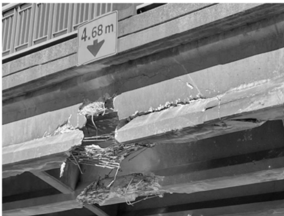
Figure 2-1 Damaged east face of Girder 5 with horizontal and diagonal web cracking
