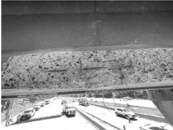
Figure 2-5 Partially Severed Tension Reinforcement and Spalling in the Bottom Flange of Girder 3 (West Face)
