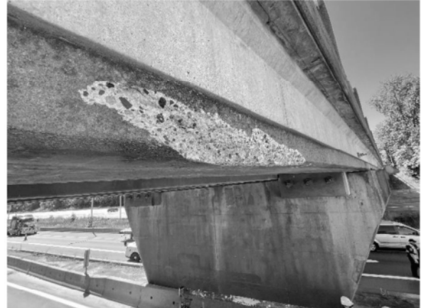
Figure 2-8 Spalling in the Bottom Flange of Girder 1 (West Face)
