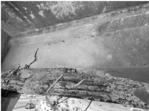
Figure 2-3 Damaged/Severed Tension Reinforcement and Diagonal/Horizontal Cracking in the Web of Girder 4 (East Face)
