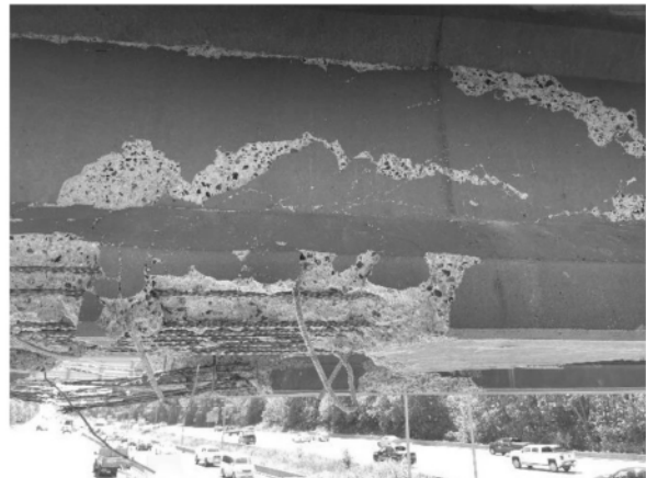
Figure 2-4 Spalling and Diagonal/Horizontal Cracking in the Web of Girder of Girder 4 (West Face)
