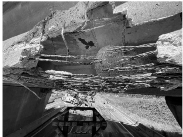
Figure 2-2 Broken reinforcement and spalled concrete at Girder 5
