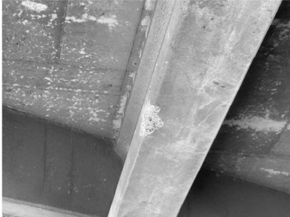
Figure 2-7 Minor Spalling in the Bottom Flange of Girder 2 (East Face)
