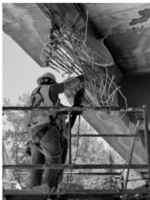
Removal of girder reinforcing and other loose debris.
