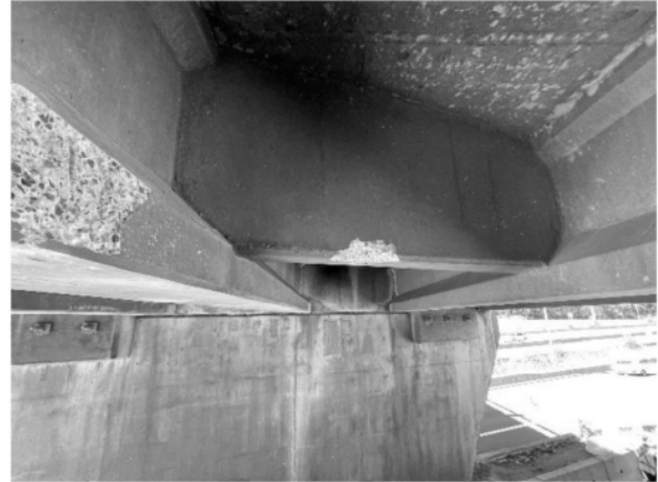
Figure 2-6 Spalling at Bottom of the Diaphragm Between Girder 2 and Girder 3 (North Face)
