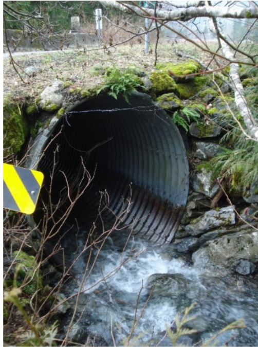
Figure 2-8 Kosikar Road 2100 mm Diameter Culvert Inlet
