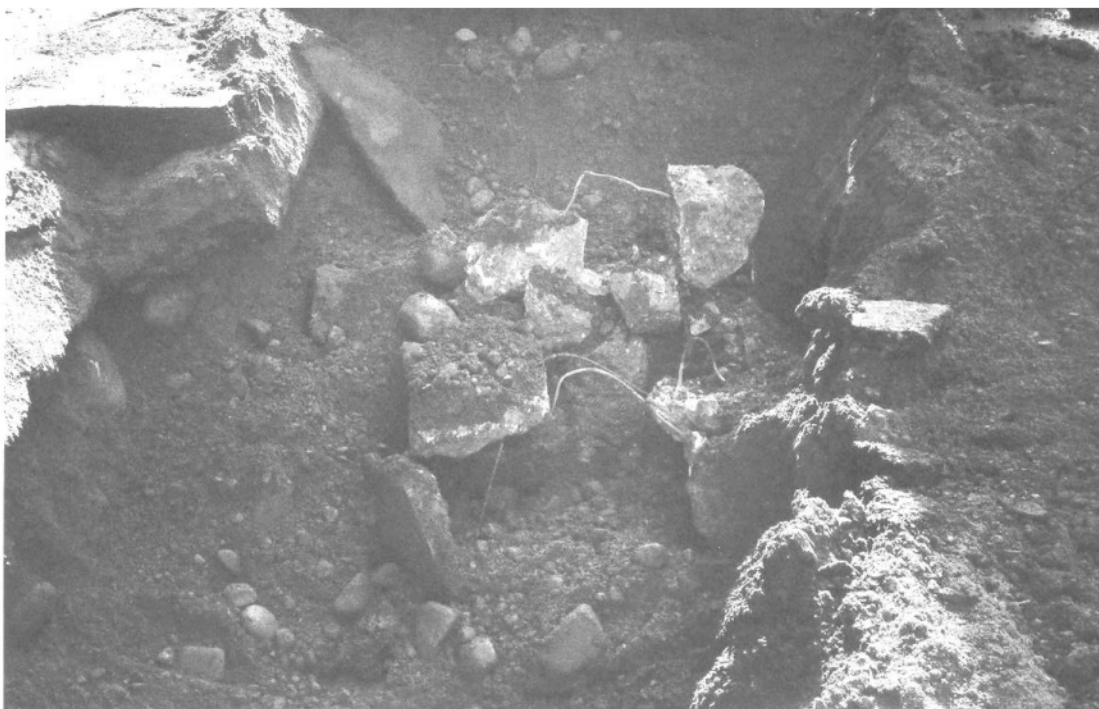
PHOTO 7: Debris, including concrete and asphalt, encountered directly beneath asphalt, during initiation of 22,730 L waste oil UST excavation (October 11, 2001).
