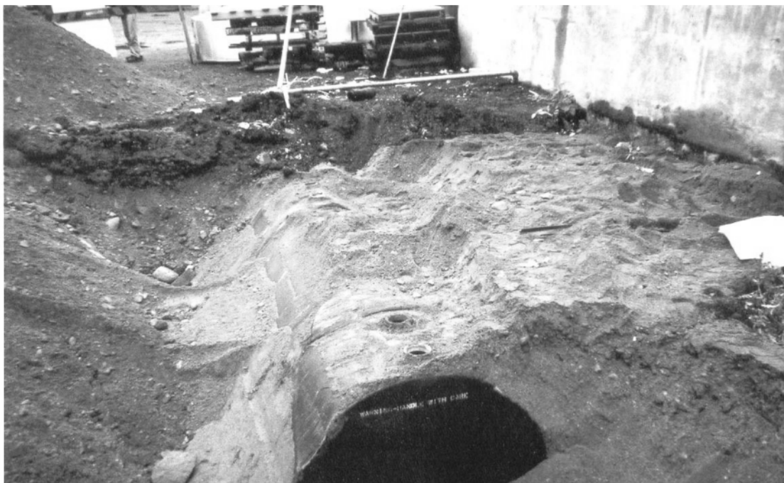
PHOTO 1: Decommissioning of 5,000 L waste oil UST (October 10, 2001). Note proximity of top of tank to ground surface (approximately 0.3 m).
