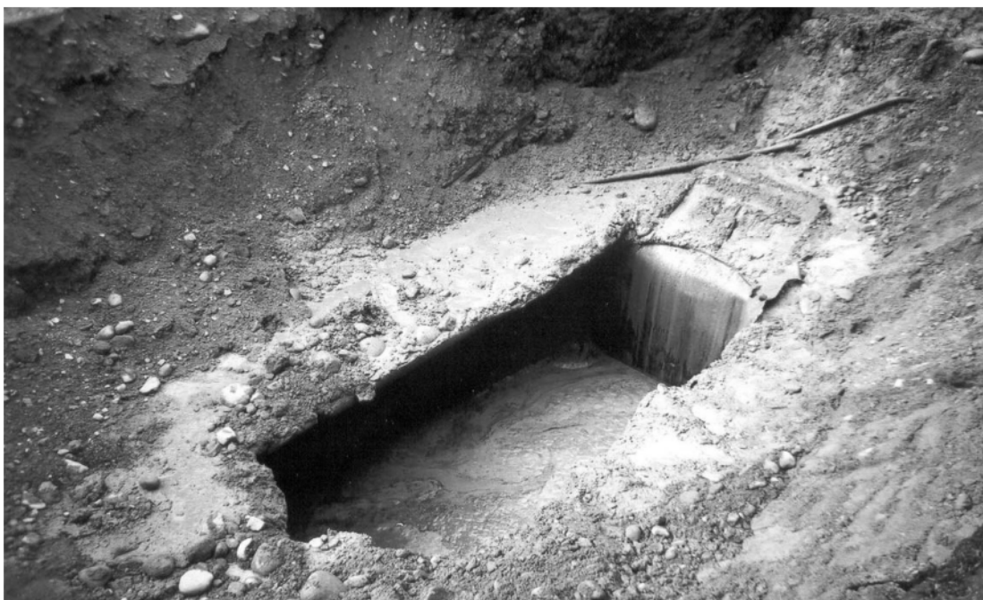
PHOTO 8: Hole cut in top of 22,730 L waste oil UST, encountered 1.8 m below ground surface. Note extensive groundwater and hydrocarbon sheen within UST.
