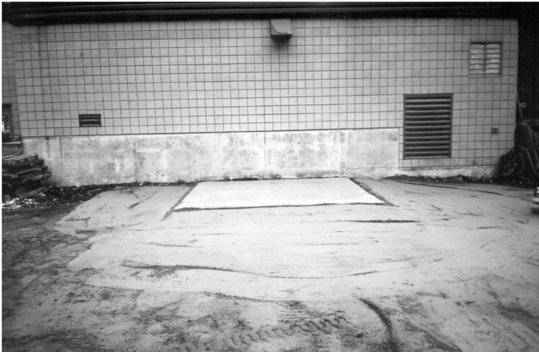
PHOTO 4: Re-instatement of 5,000 L waste oil UST excavation area with new concrete slab, facing southeast.
