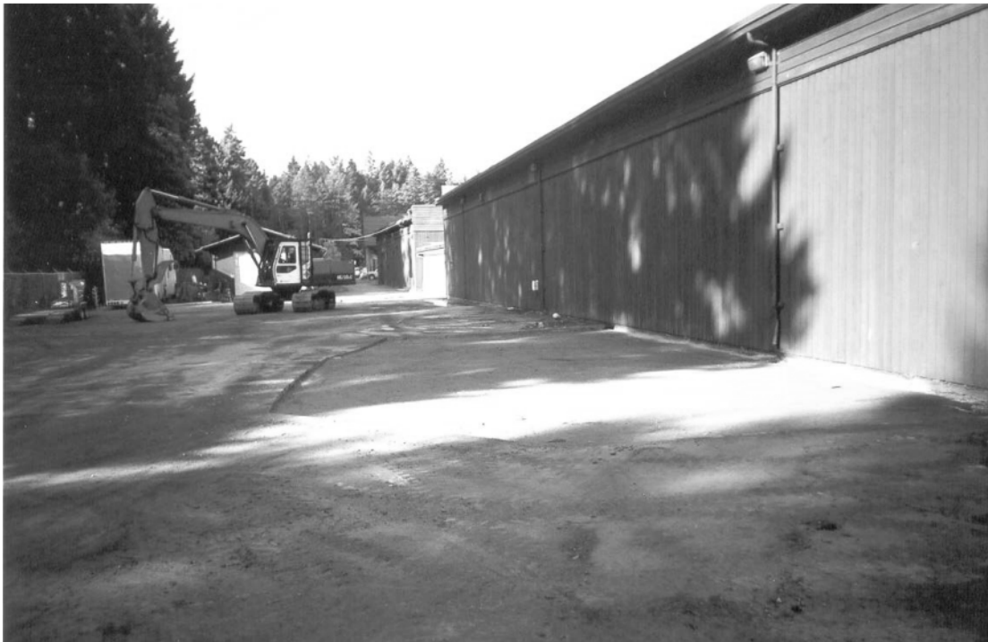
PHOTO 11: Re-instatement of 22,730 waste oil UST excavation area, prior to asphaltting.
