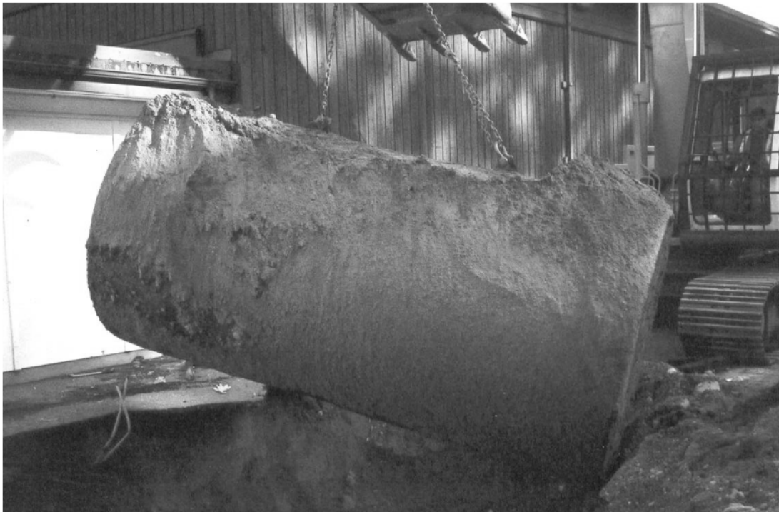
PHOTO 5: Removal of 9,100 heating oil UST (October 11, 2001).
