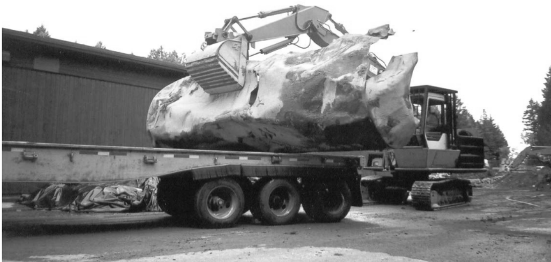
PHOTO 10: Remains of 22,730 L waste oil UST loaded onto flatbed for off-site disposal. Tank was extensively damaged during removal due to logistical difficulties.
