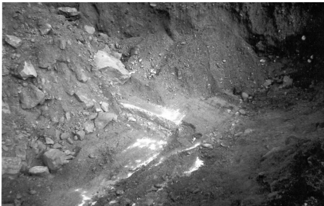
PHOTO 2: Concrete slab below 5,000 L waste oil UST. Note bedrock subcrop directly beneath concrete slab.
