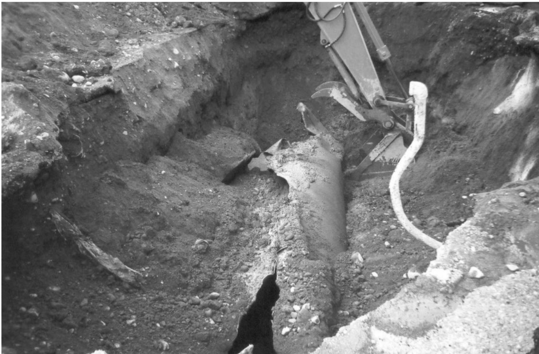
PHOTO 9: Removal of 22,730 L UST (October 12, 2001). Note former vent pipe in foreground.
