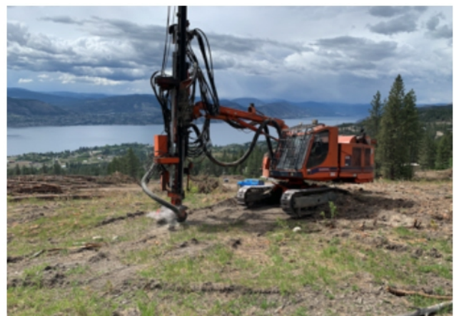
Photo 12: Typical drill probing for bedrock
