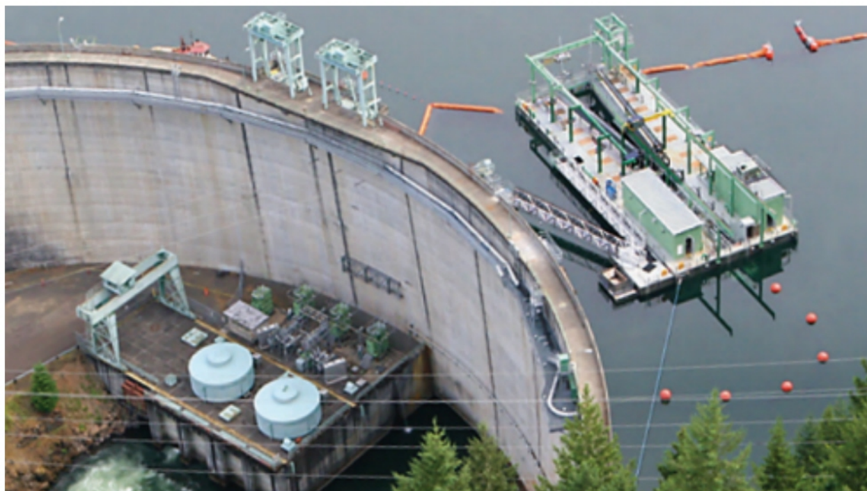
Figure 4-4 Floating Surface Collector at North Fork on the Clackamas River, PGE
