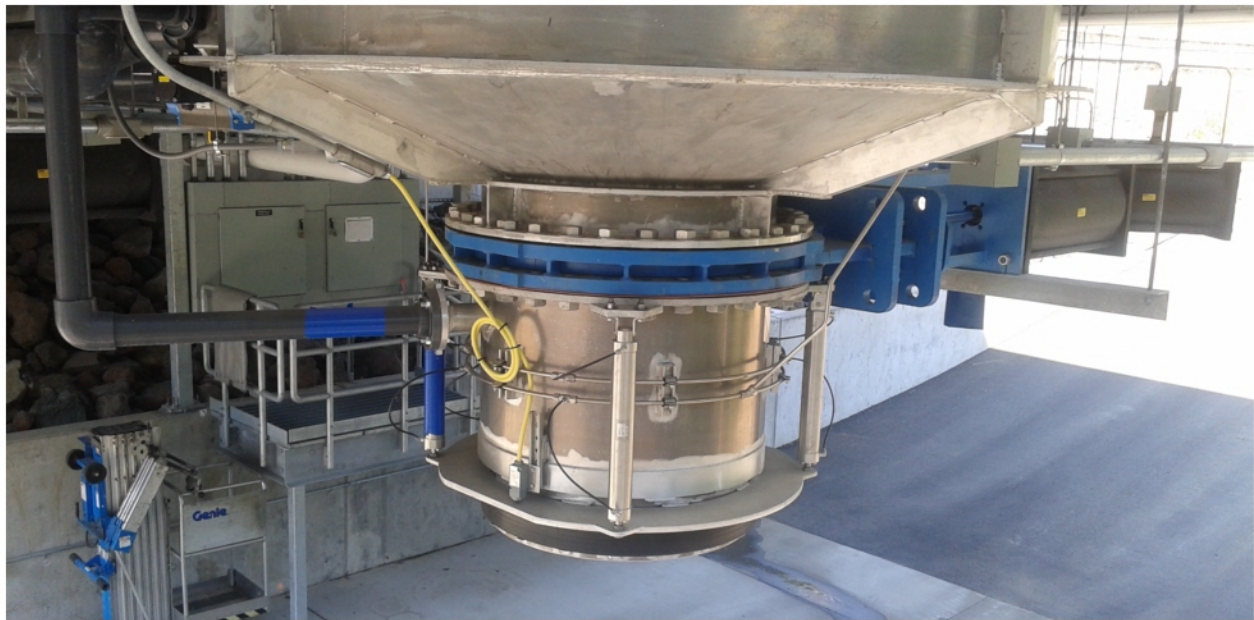
Figure 4-3. Example of Valve Allowing the Water-to-Water transfer (e.g., Clackamas Adult Collection Facility)
