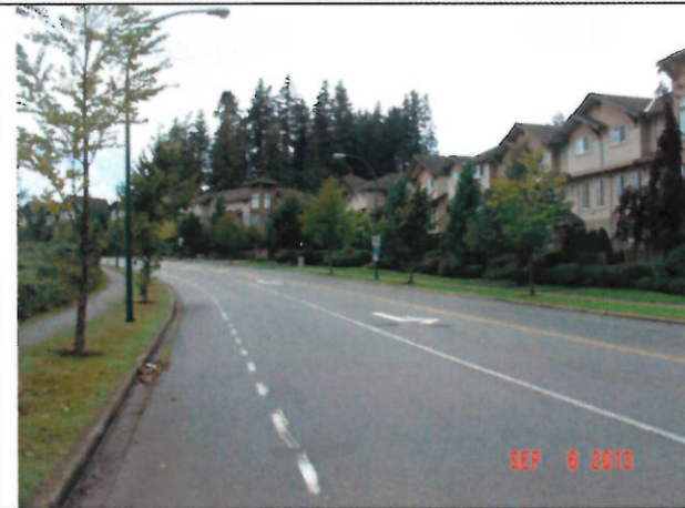
Panorama Drive – Facing west
