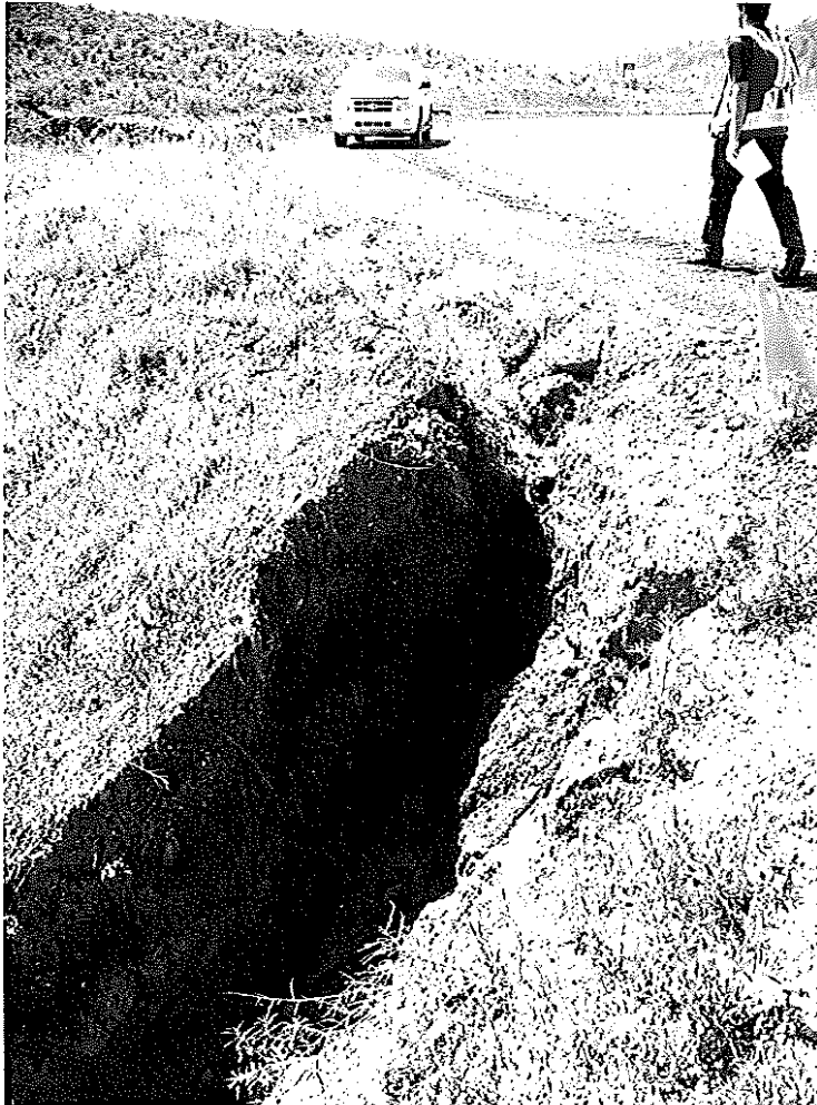
Photo 1: Improper Roadside Drainage Apron
