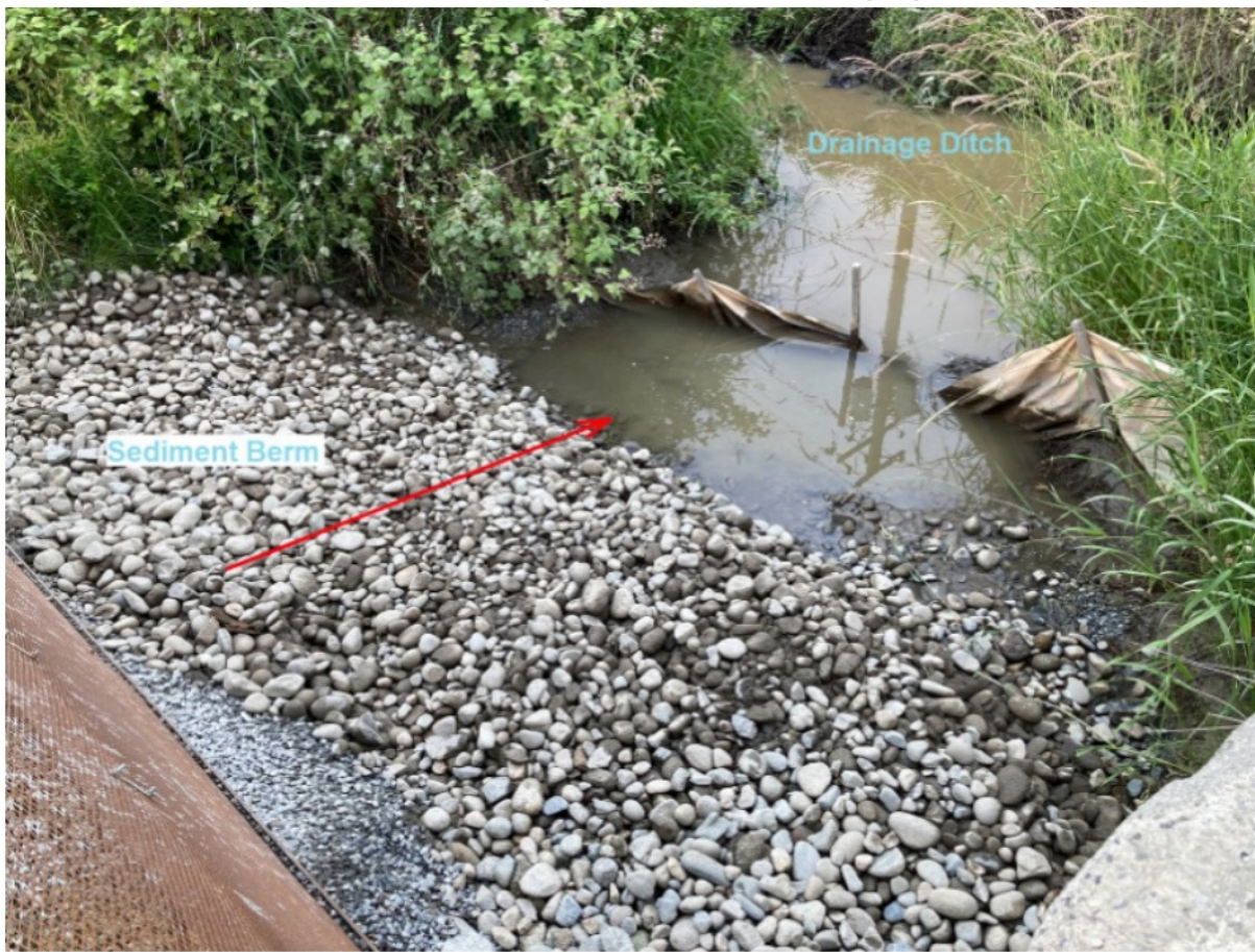
Attachment 5: Photo 4 North Drainage swale to ditch through gravel berm.
