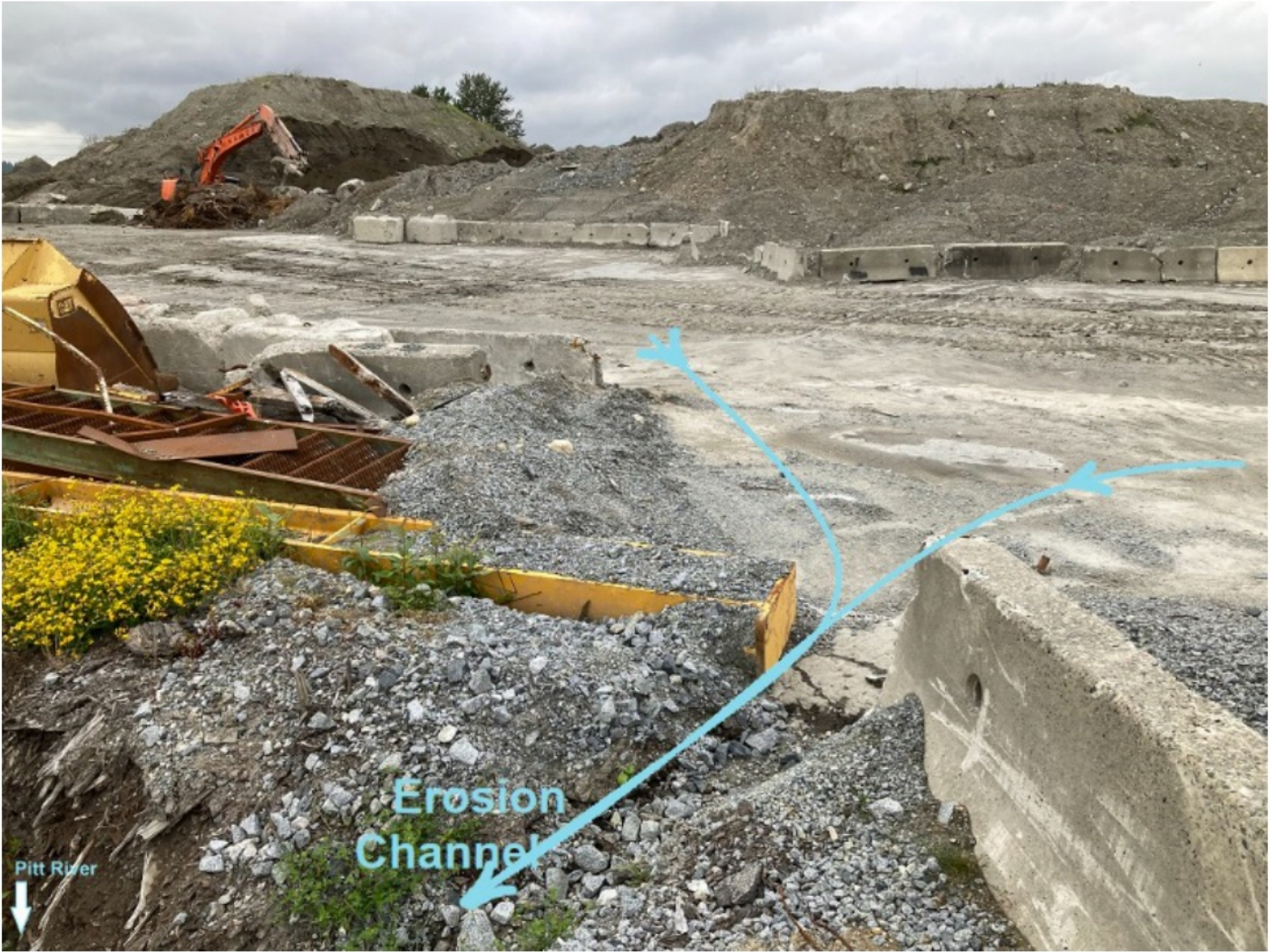
Attachment 4: Photo 3 Erosion channel to Pitt River
